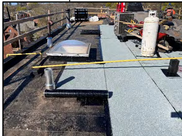
Installation of New Modified Bitumen Cap Sheet
