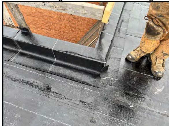
Installation of New Insulation, Modified Bitumen Roofing & Membrane Flashings
