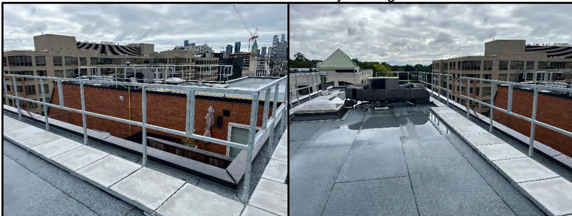
Installation of New Safety Railings
