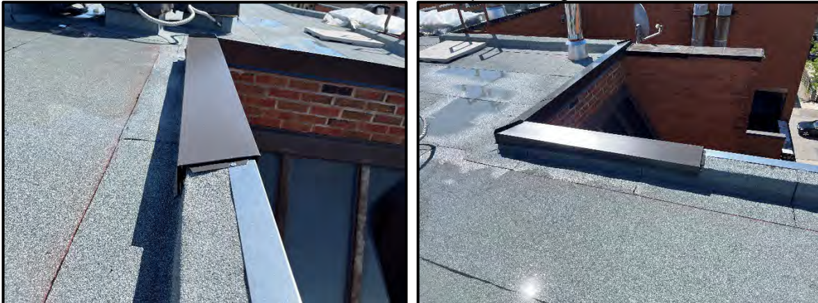
Installation of Metal Cap Flashing
