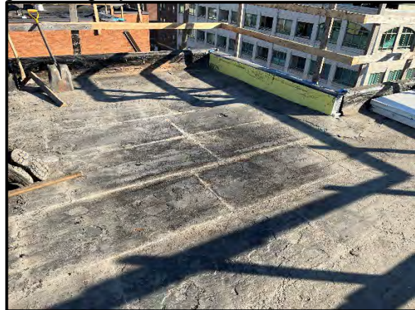
Removal of Existing Roofing System
