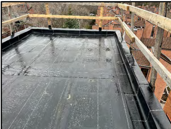
Installation of New Insulation, Modified Bitumen Roofing & Membrane Flashings
