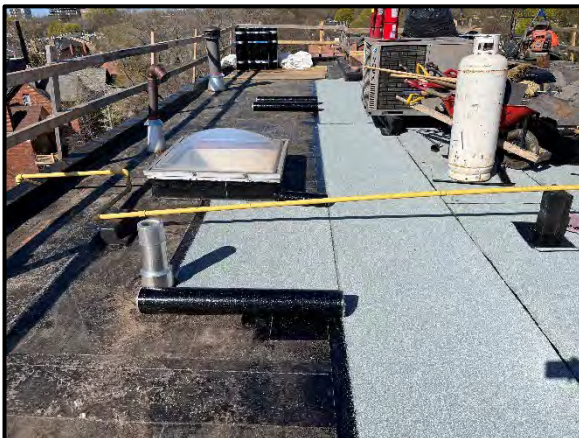
Installation of New Modified Bitumen Cap Sheet
