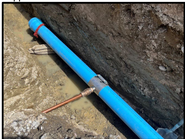
Installation of new PVC watermain and copper water service
