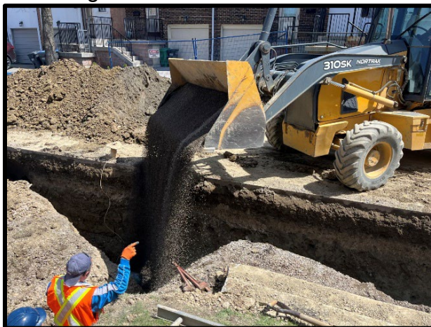
Backfilling the excavated trench
