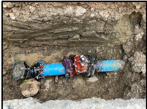
Installation of new gate valve
