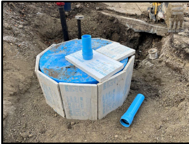
Installation of new precast concrete chamber
