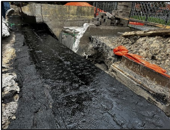
Local garage slab waterproofing membrane replacement at garage roof slab down-turns
