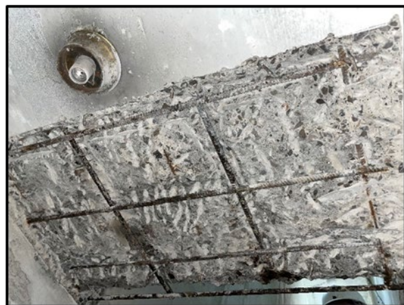
Localized underside (soffit) concrete repairs
