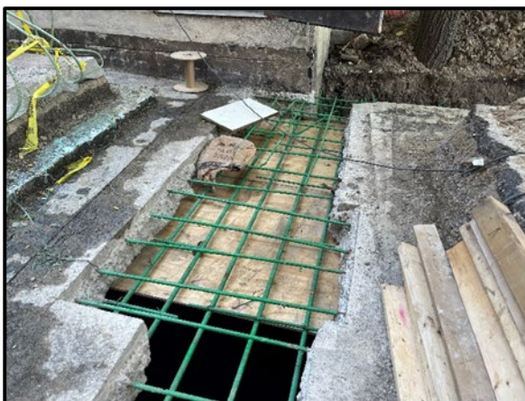
Localized through-slab concrete repairs
