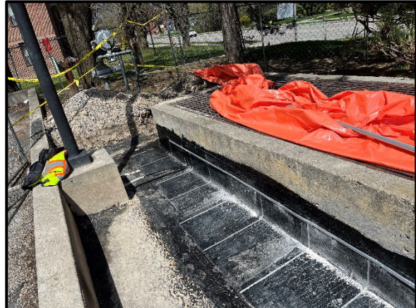
Local garage slab waterproofing membrane replacement at garage roof slab up-turns
