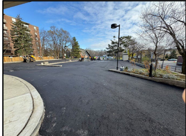
Installation of new asphalt pavement surface course.
