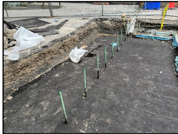
Localized waterproofing membrane replacement at garage roof slab field areas
