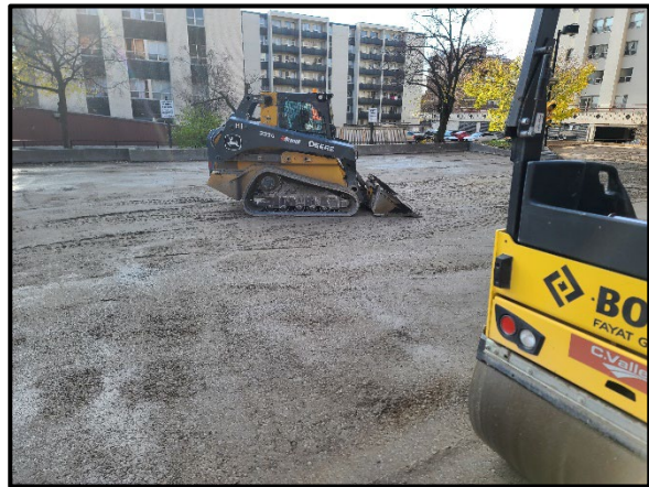
Installation of new granular base at parking lot
