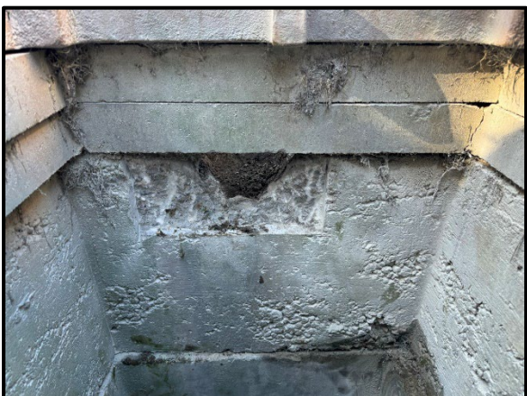
Localized repairs to the west catch basin
