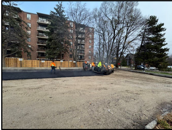
Installation of new asphalt pavement binder course.
