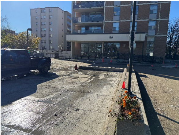
Asphalt pavement removals at parking lot
