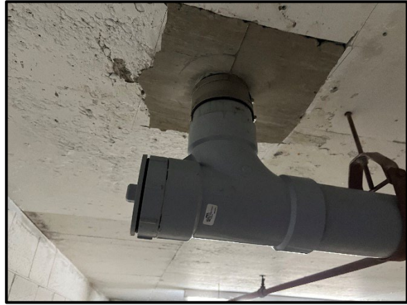
Localized roof slab drainage piping replacement
