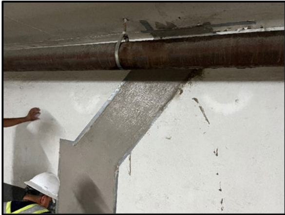
New cementitious capillary crystalline waterproofing at garage walls
