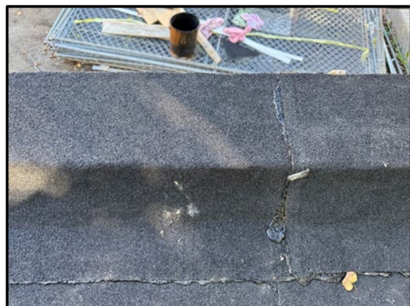
Garage exit stairwell flat roofing system replacement
