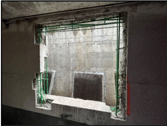
Localized vertical surface concrete repairs
