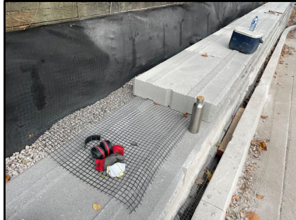
Geogrid reinforcement installation at modified section of the wall
