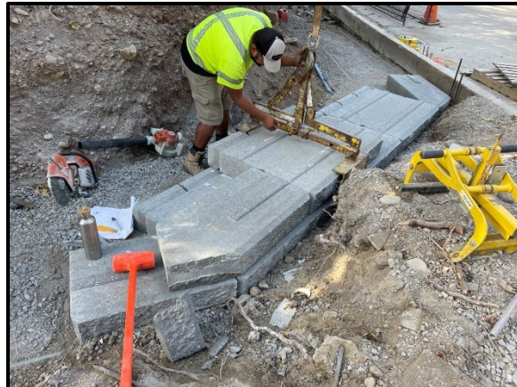
Installation of retaining wall base stones
