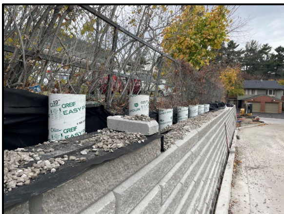
Installation of fence post forms
