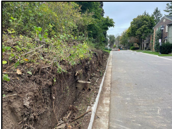
Installation of U-fill base
