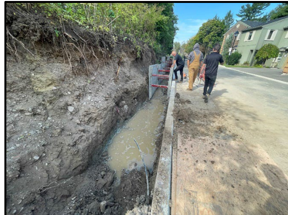
Installation of U-fill base
