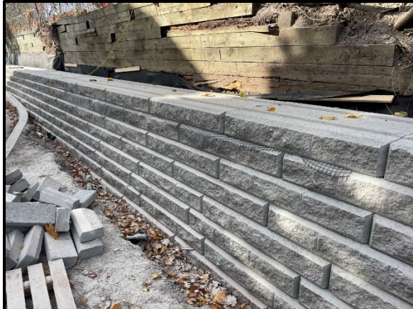
Installation of retaining wall stones
