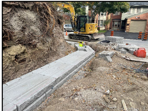
3/4" clearstone backfill with filter cloth
