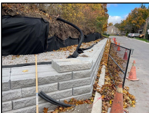
3/4" clearstone backfill with filter cloth
