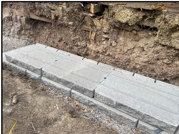
3/4" clearstone backfill with filter cloth
