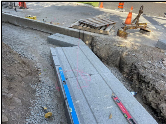
Installation of retaining wall base stones
