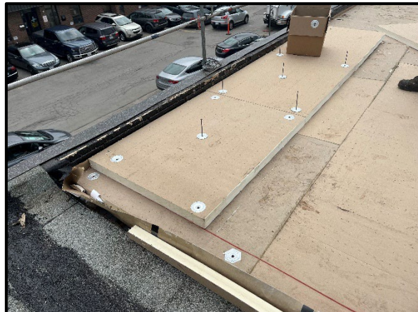
New roof insulation
