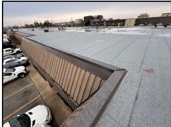
New metal perimeter flashings
