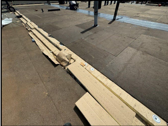
New substrate board
