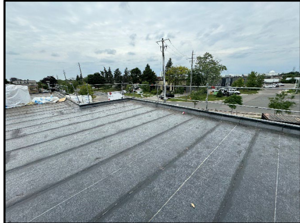
New base sheet membrane
