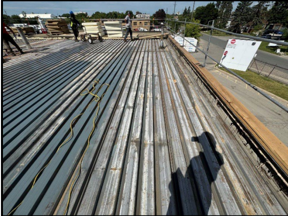
Local cleaning and recoating of the existing steel deck
