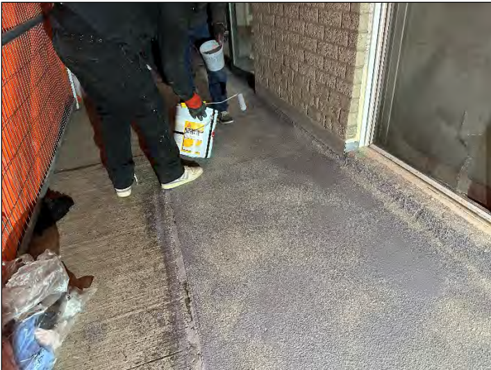
Garage Roof Slab Waterproofing
