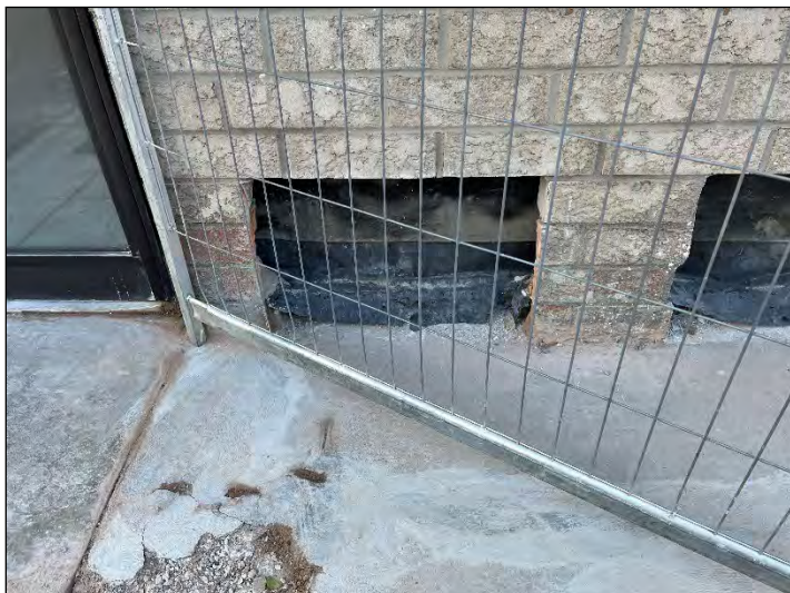
Localized Concrete Removal
