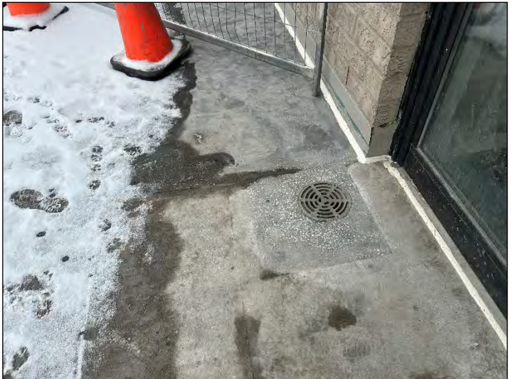
New Drain Installation
