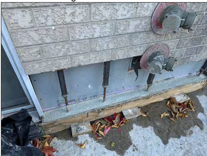
New Sheathing and Concrete Curb Installation
