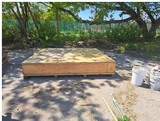
Photo #5- Waterproofing membrane at top of Mosaic Knob Hill Farm Logo skid was not installed, to be reviewed by Heritage Architect for further comments
