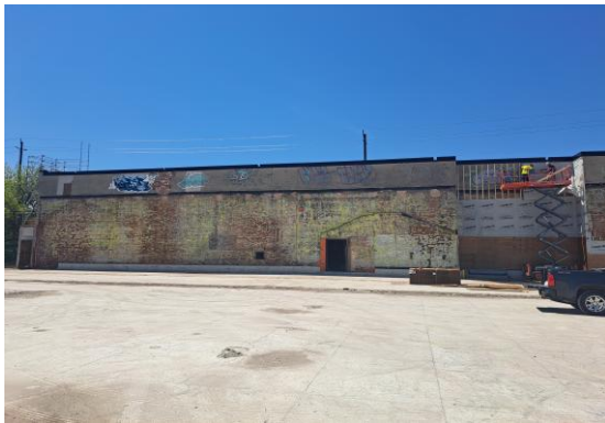
Photo #1- Installation of pressure treated plywood for weather proofing of part 1 building on the east side was underway, to be reviewed by Heritage Architect for further comments.
