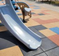
3. Level tiles to remove exposed edge and obtain a smooth surface. Two areas identified include below the rope climber and adjacent the southernmost shade post.
