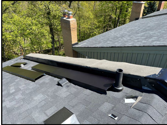
Bonded underlayment at firewalls
