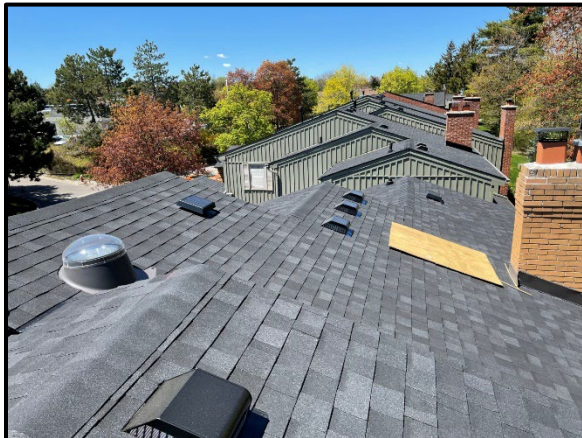
Installation of new roof vents
