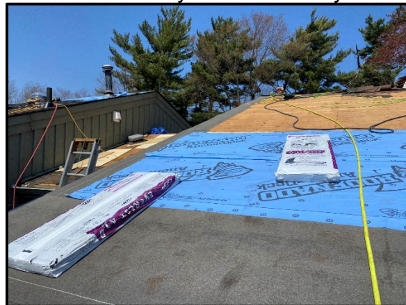
Installation of Synthetic Underlayment
