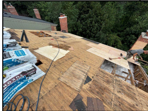
Replacement of deteriorated sheathing
