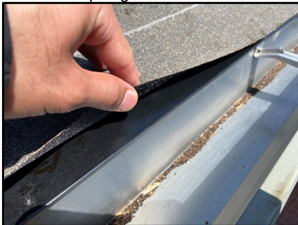
Metal drip edge installation at eaves
