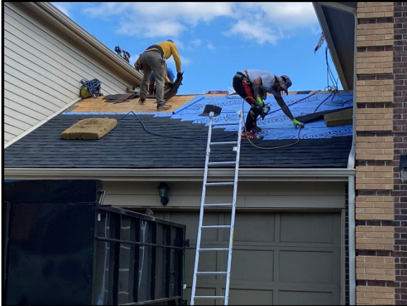
Asphalt Shingle installation
