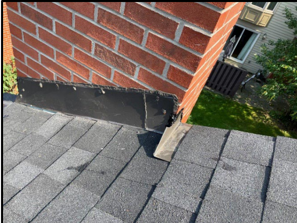
Metal counterflashing installation
