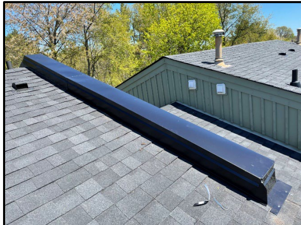
Metal Flashing at firewalls
