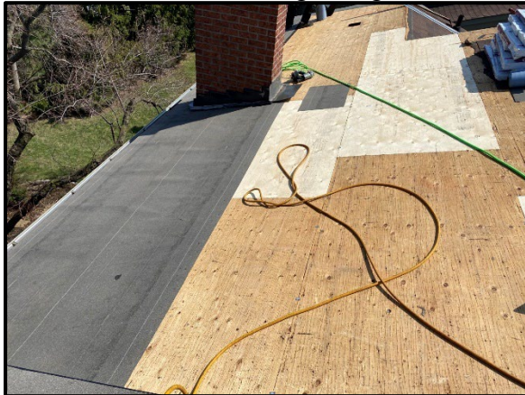
Removal of existing shingles
