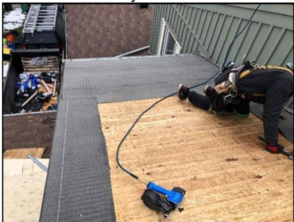
Bonded underlayment for 6' at eaves
