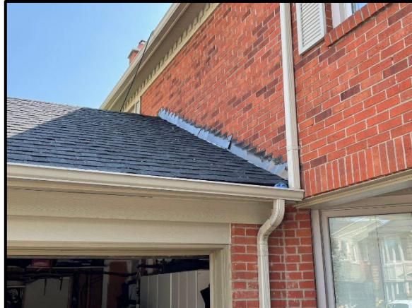
Metal counterflashing installation
