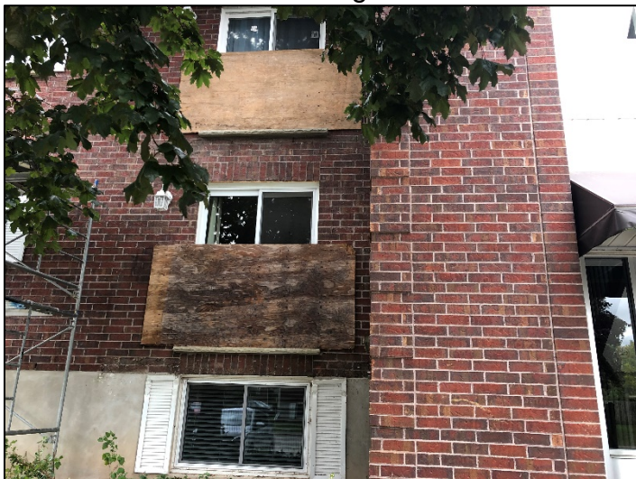
Removal of Existing Balconies
