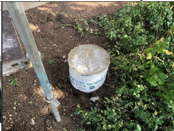
Replacement of Concrete Footings
