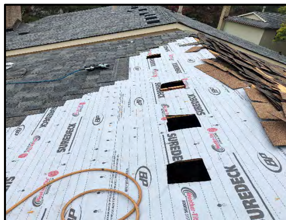
Installation of new asphalt shingles at upper and lower roofs
