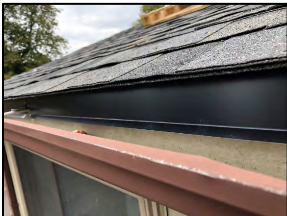
Installation of Metal Drip Edge at eaves and rakes
