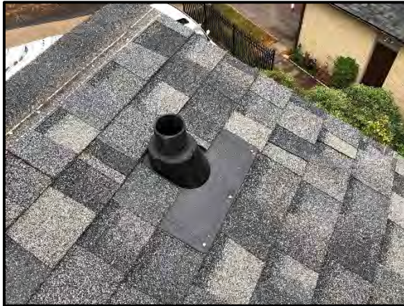
Installation of new asphalt shingles at upper and lower roofs
