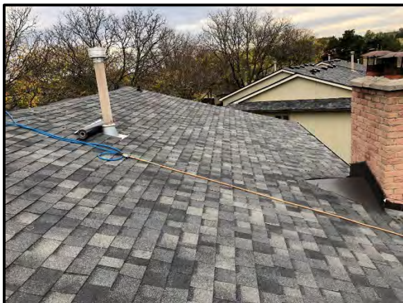
Installation of new asphalt shingles at upper and lower roofs
