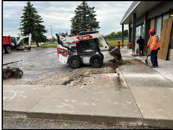
Removal of concrete for barrier free curb ramps
