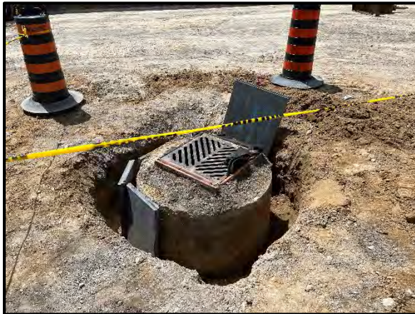
Installation of insulation around catch basin
