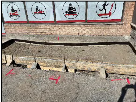
Forming of barrier free curb ramps
