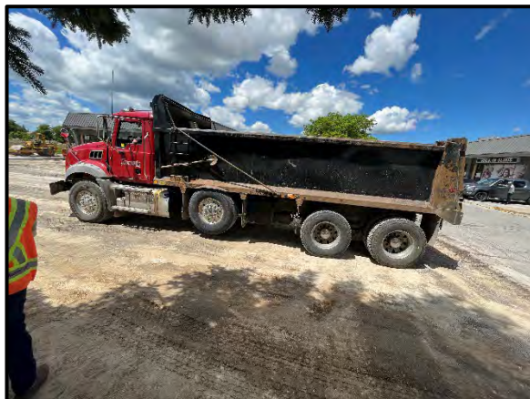
Proof rolling of existing granular subgrade
