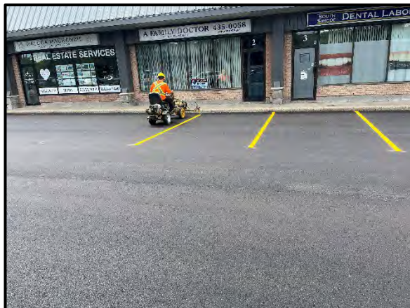
Installation of pavement markings
