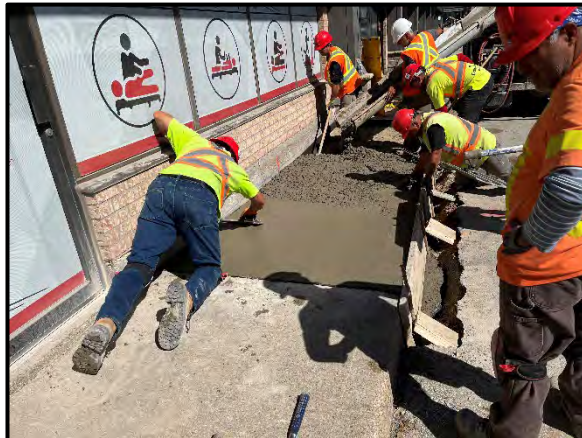
Placement of concrete at barrier free curb ramps
