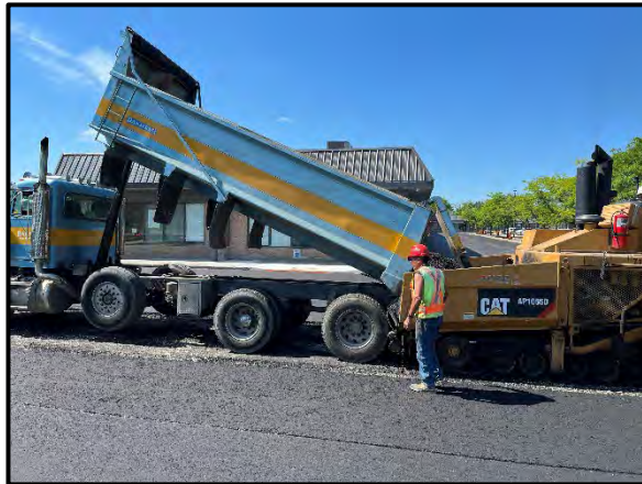
Placement of binder course asphalt
