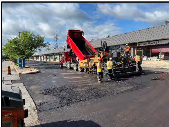
Placement of surface course asphalt
