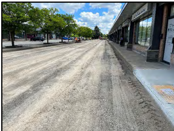
Removal of asphalt in the 'Phase 1' areas
