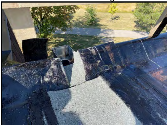
Installation of self-adhered modified bitumen base sheet flashing.
