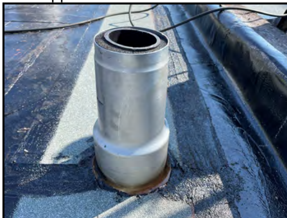
Installation of metal stack flashings and torch applied base sheet membrane.
