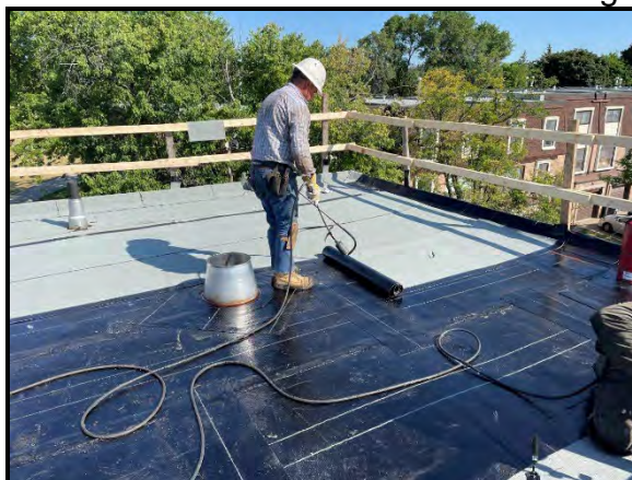
Installation of the torch-applied modified bitumen base sheet membrane flashing.
