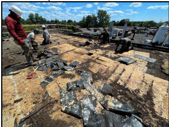
Removal of the existing flat roofing and related components.
