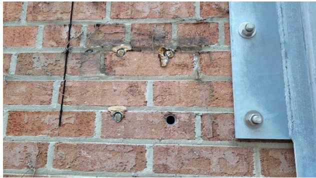
Photo 8: Contractor to infill voids leftover from existing steel framing removal with sealant.
