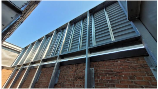
Photo 6: Steel framing was found to be installed. No brick were found to be damaged. Work was found to be acceptable.
