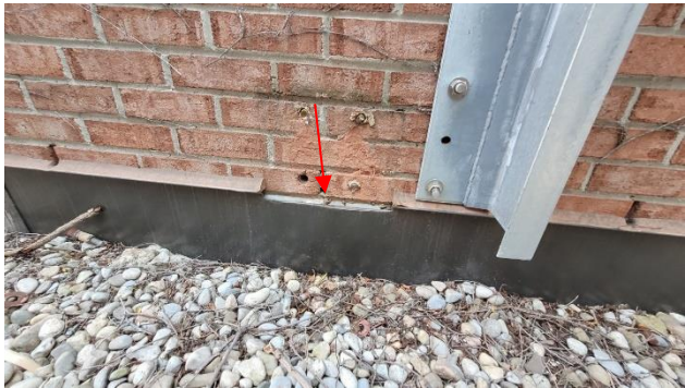
Photo 7: Contractor to caulk the top of the wall upturn metal flashing to ensure watertight seal.
