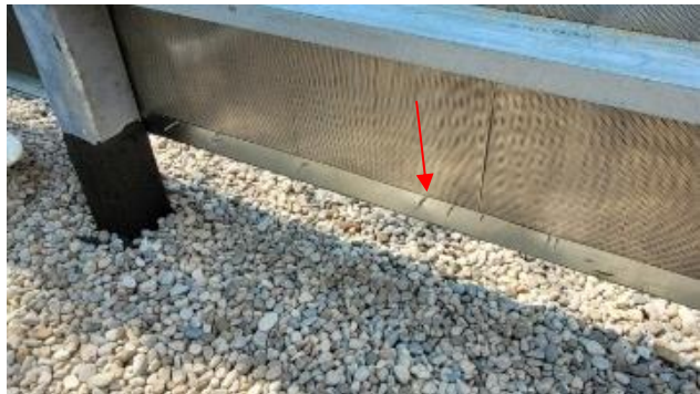
Photo 10: Contractor to grind the ends of the fasteners to create a blunt end.
