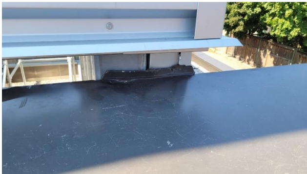
Photo 9: Contractor to apply sealant at parapet cap flashing to steel framing junction.
