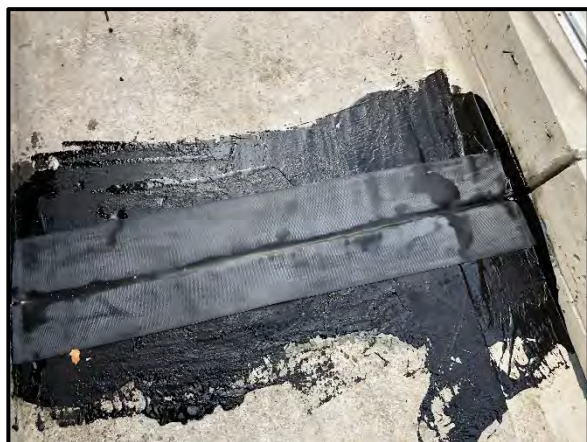
Installation of hot-applied waterproofing membrane at expansion joints.
