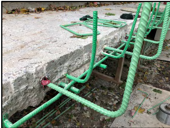
Installation of new concrete beam.
