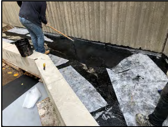
Installation of modified bitumen base sheet, metal fastening bars and protection board.
