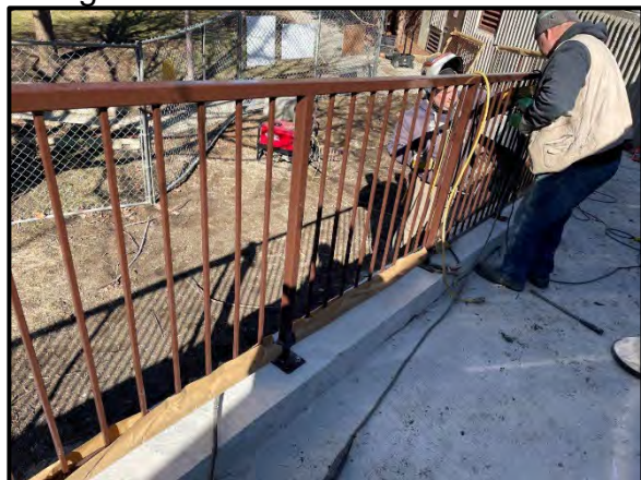
Installation of pre-painted galvanized steel railings.
