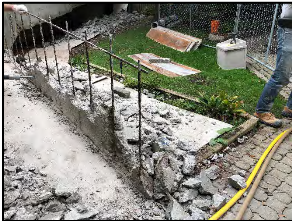
Installation of new pre-epoxy coated reinforcement bars.
