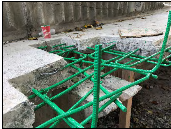
Installation of formwork to facilitate installation of new concrete beam.
