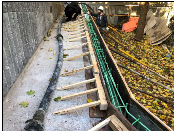
Installation of hot-applied waterproofing membrane at expansion joints.
