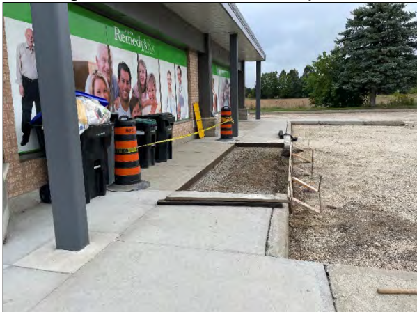
Forming of barrier free curb ramps
