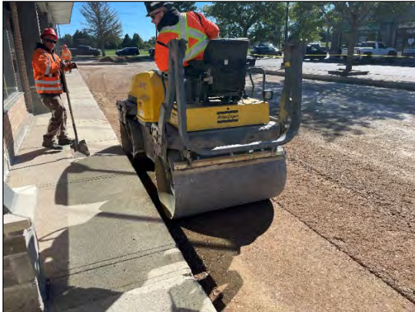
Granular replacement and compaction
