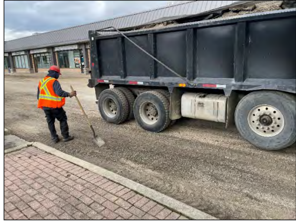
Existing granular base proof rolled
