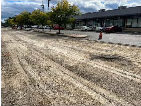
Existing asphalt removal
