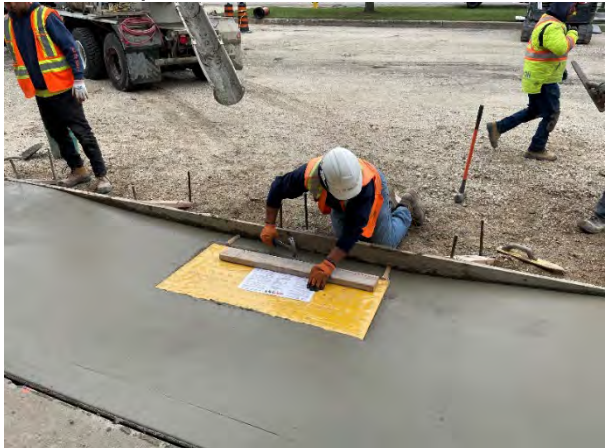
Concrete placement at barrier free curb ramps
