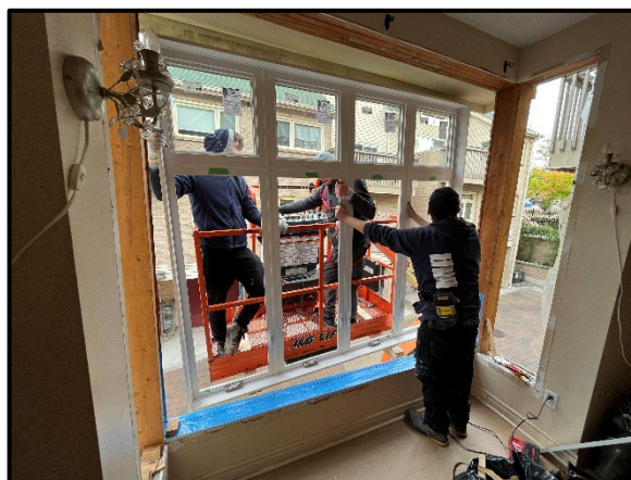
Installation of new vinyl windows.
