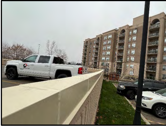
Installation of metal cap flashing
