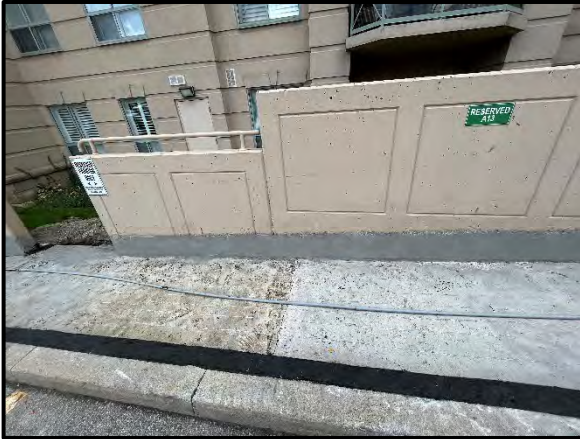
Concrete preparation to wall upturn (Above stall Nos. 66-74)
