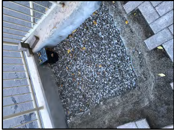
Installation of new garage roof slab drain (Below the pedestrian ramp)
