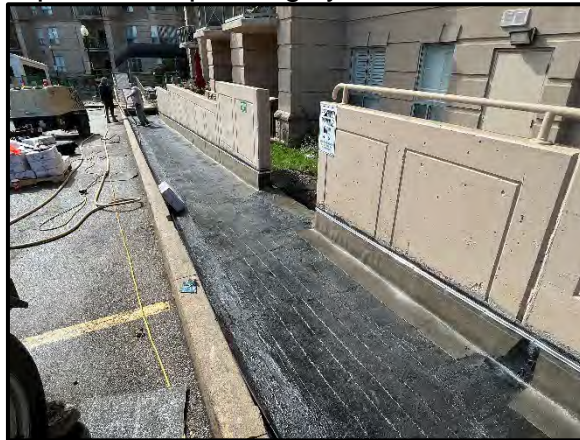
Installation of hot-applied rubberized asphalt waterproofing system
