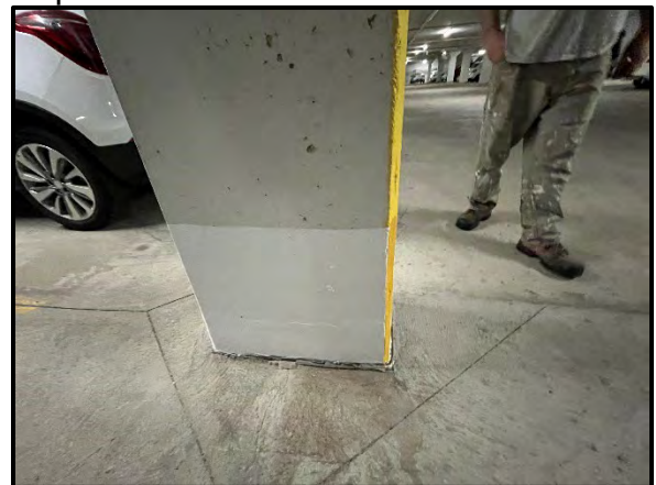
Repaired column bases
