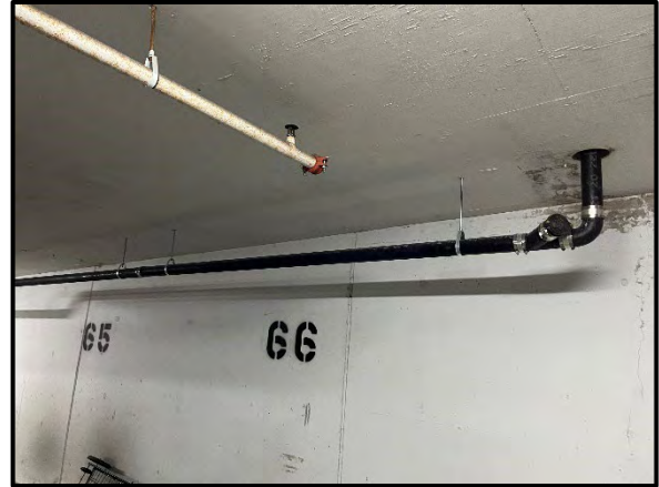
Installed garage roof slab drain pipe (South end of the site wall)
