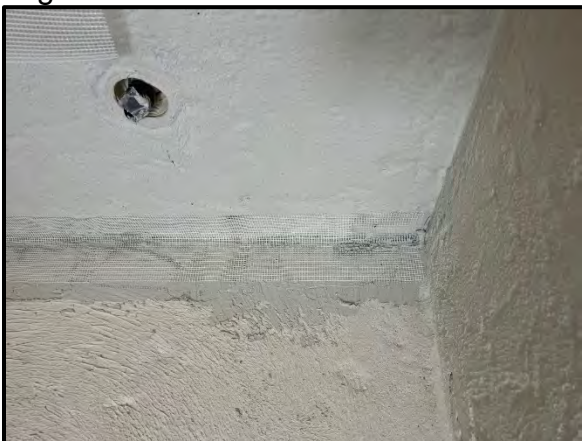
Reinforcement mesh embedded into the Tapecrete top coat, at the corners and edges of the basin.
