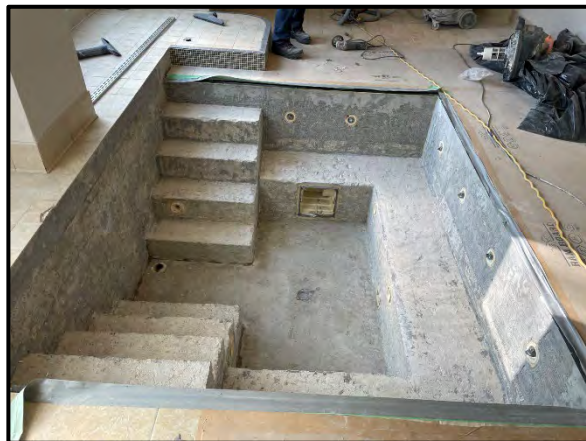
Whirlpool basin concrete surface prep.
