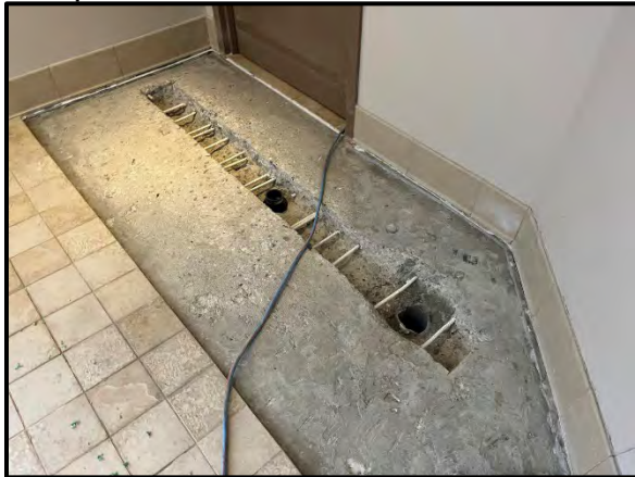
Removal of floor tiles and concrete around existing floor drains on either side of the whirlpool room.
