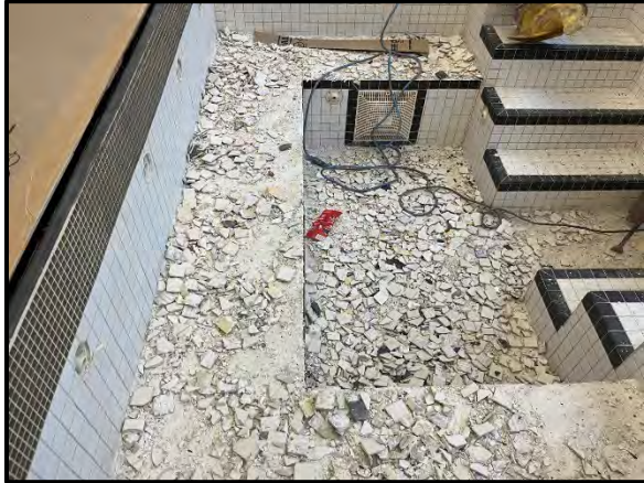
Removal of existing whirlpool basin tiles.
