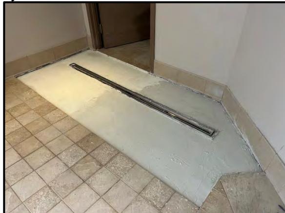
Installation of the Tapecrete waterproofing system around the new linear drains.
