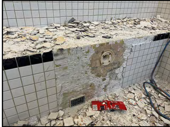
Removal of existing whirlpool basin tiles.
