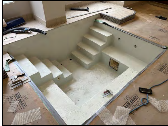
Installation of the Tapecrete waterproofing system top coat in the whirlpool basin.
