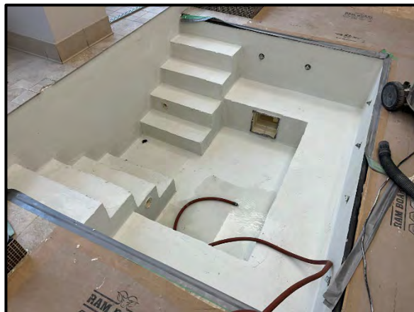
Installation of the Tapecrete waterproofing system around the new linear drains.
