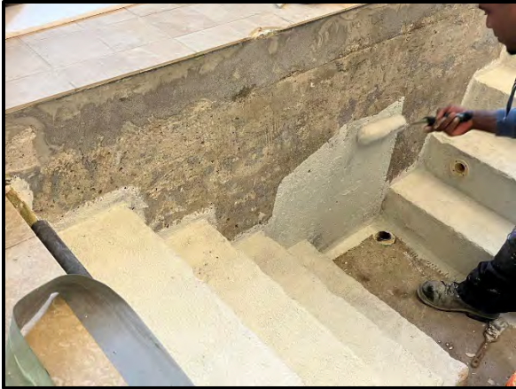
Installation of the Tapecrete waterproofing system base coat in the whirlpool basin.
