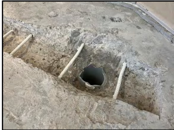
Whirlpool basin concrete surface prep.
