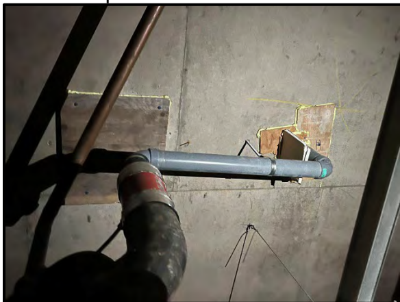
Installation of new drainpipes on either side of the whirlpool room.
