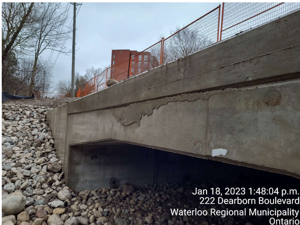
Photograph 2: View of the concrete overpour on the south fascia
