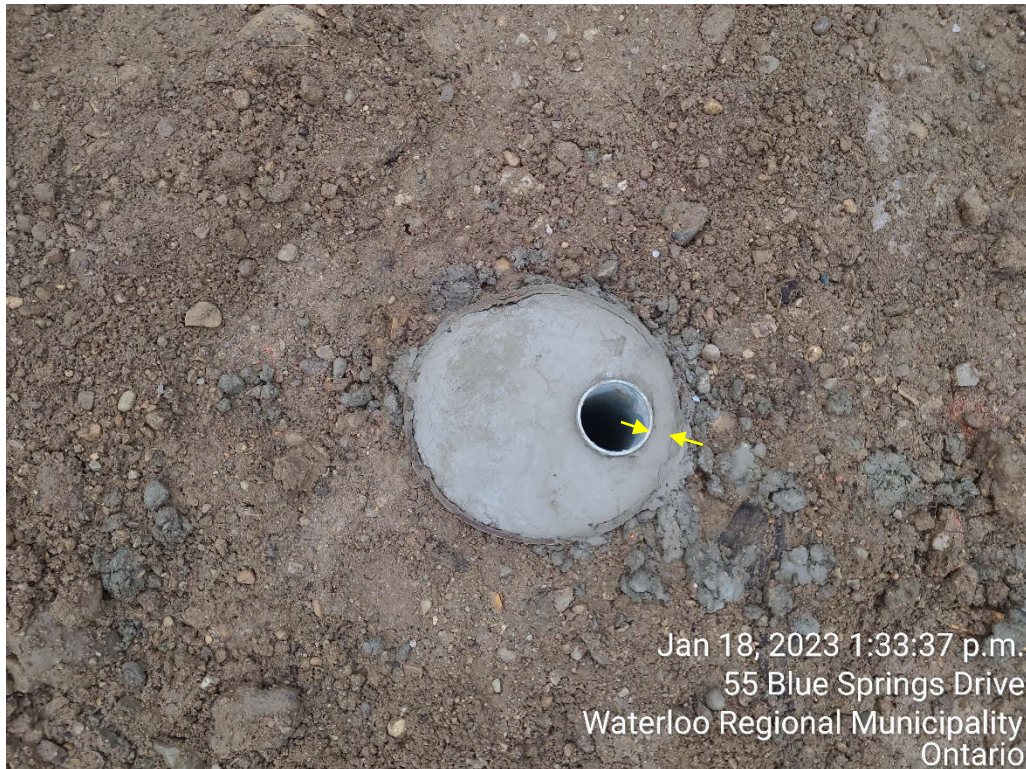
Photograph 1: Typical railing base with insufficient concrete cover on the steel sleeve
