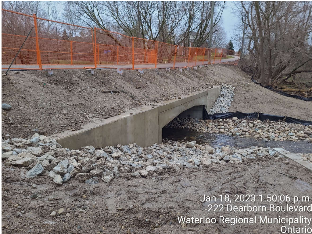
Photograph 7: Typical area requiring restoration on the downstream side of the structure
