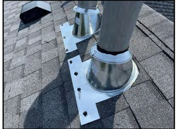
New chimney base and collar flashings.
