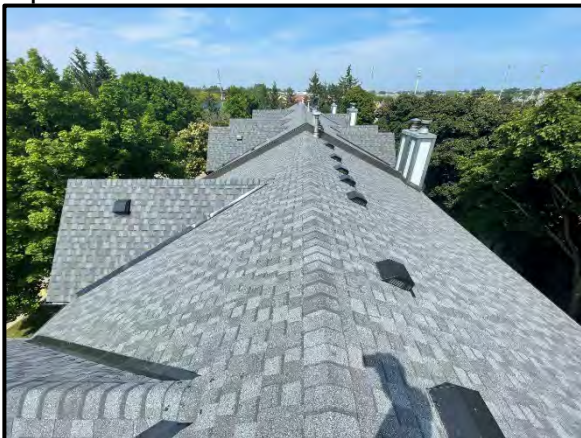
Completed asphalt shingle roofing replacements.
