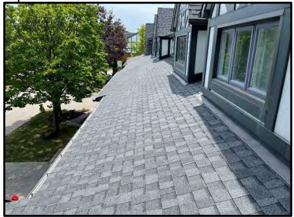
Completed asphalt shingle roofing replacements.
