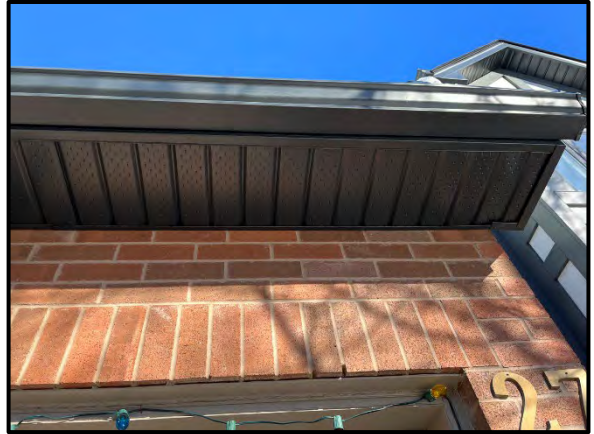
Installation of new perforated aluminium soffits.
