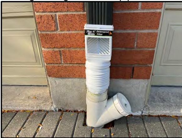
Installation of new PVC downspout filters at the ground level including connection into existing underground drainpipes
