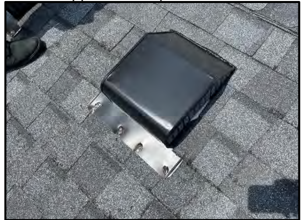
Installation of six (6) new roof attic vents at the rear upper roof slopes of each unit.
