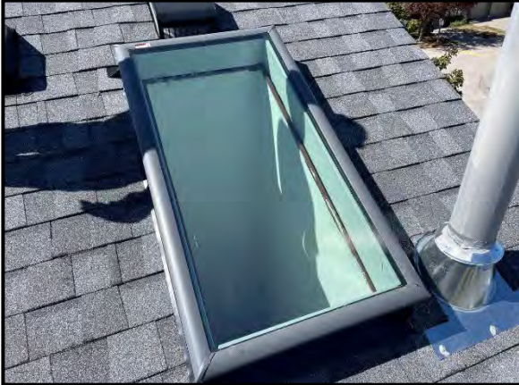
Installation of new skylights.
