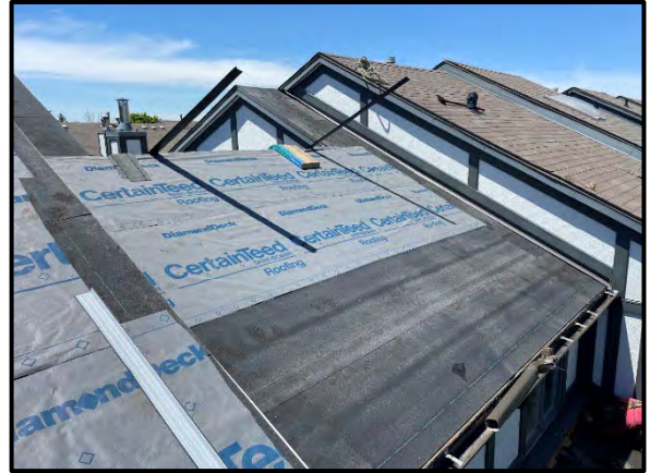
Synthetic underlayment installed at remaining upper roof exposed sheathing.
