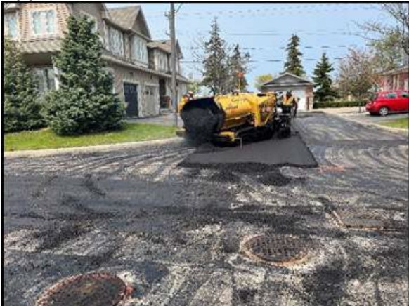
Application of tack coat
