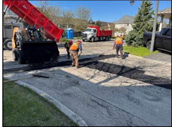
Installation of localized binder course
