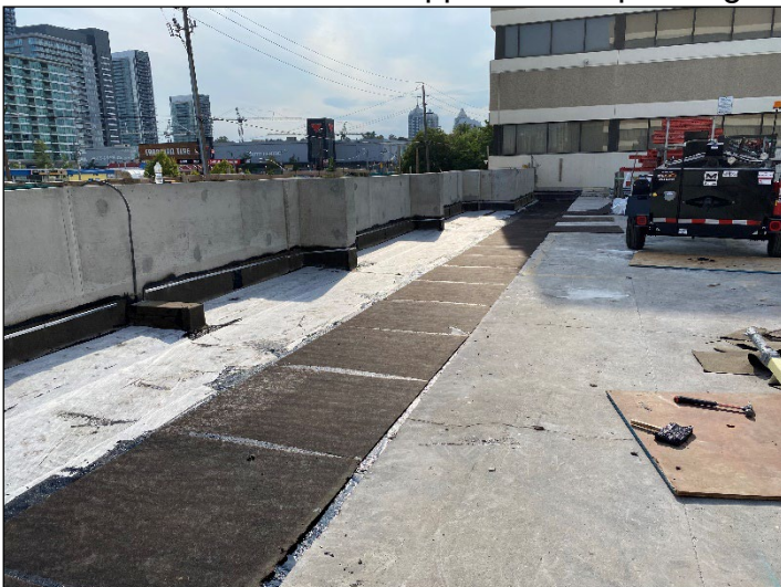
Installation of New Hot-Applied Waterproofing
