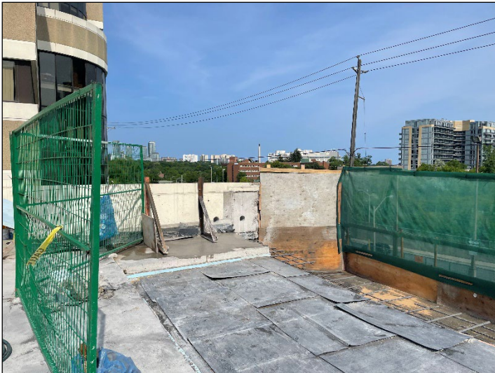
Installation of New Hot-Applied Waterproofing
