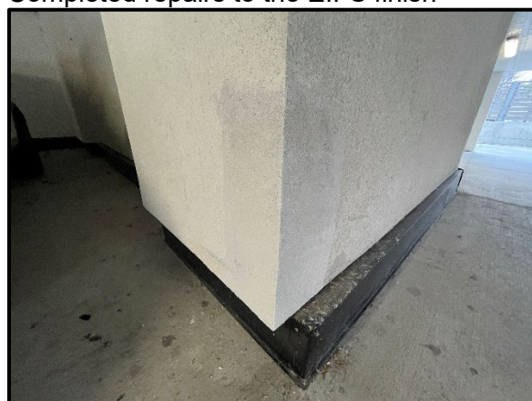
Completed repairs to the EIFS finish
