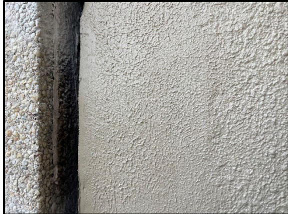
Installation of two-stage sealants at the wide exterior joints
