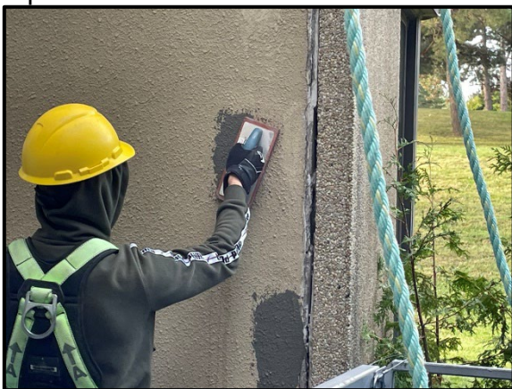
Cast-in-place vertical concrete shear wall repairs
