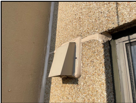
Installation of new exterior sealants
