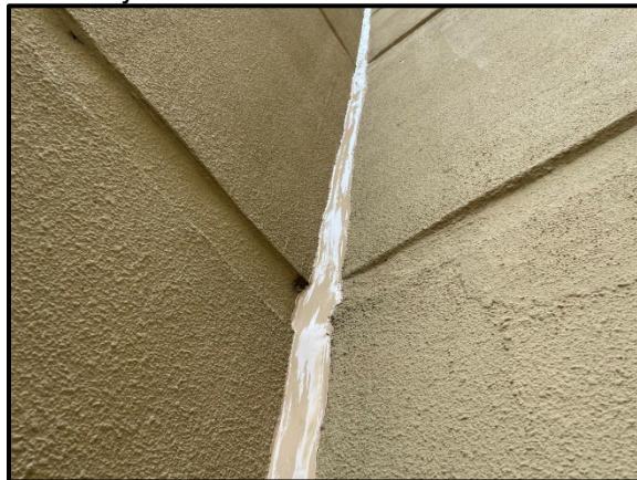
Installation of two-stage sealants at the wide exterior joints
