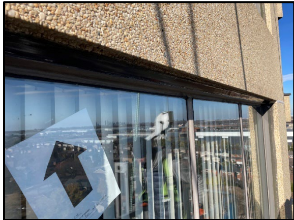
Localized replacement of window perimeter sealants
