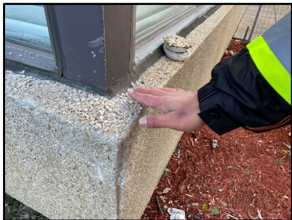
Precast wall panel repair mock-up
