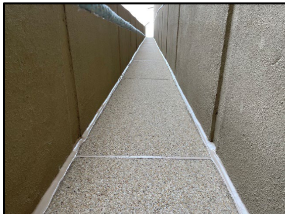
Installation of new exterior sealants
