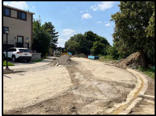
Backfilling the excavated trenches
