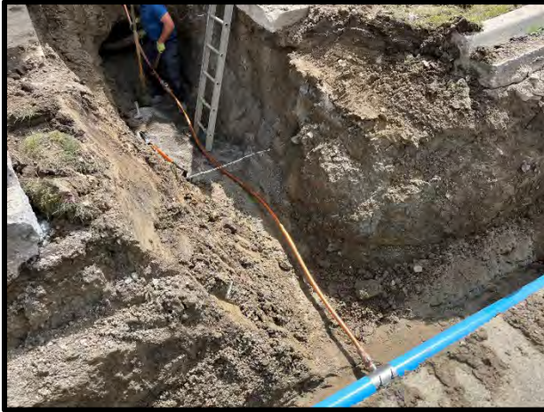
New copper water service installation
