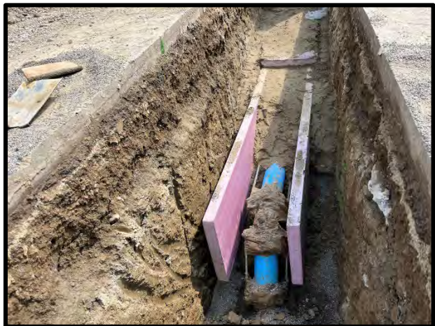
New watermain installation with related insulation details
