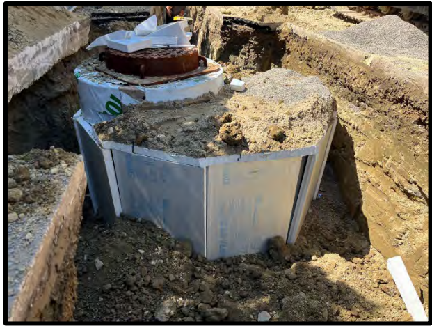
Insulation and waterproofing installation over the chamber body
