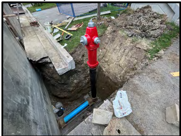
New fire hydrant installation
