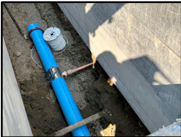
Gate valve installation
