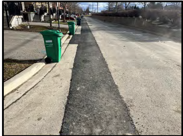
Asphalt pavement installation
