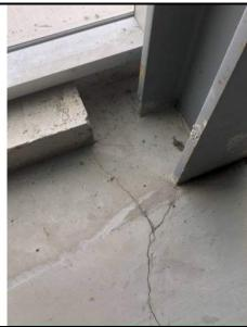
Photo 46 Floor cracking at center office area to be reviewed by Struct Eng.& installer.
