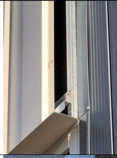
Photo 40 View at typical flashing to be completed on edge of Morin siding. Ensure envelope drains properly. & all hat bars are fully concealed.
