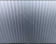
Photo 28 Scratches on North wall above sidewalk to be remediated per mfg. instructions.
