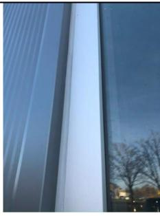
Photo 33 View of capped IMP with color matched sealant to curtainwall mullion.
