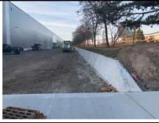
Photo 19 View at NE corner looking West. Confirm final grades will not exceed 3:1 &civil and install guard where wall exceeds 600mm in height.
