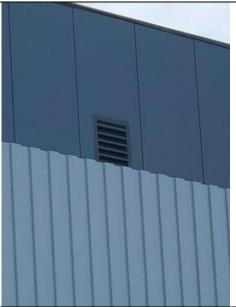
Photo 35 View looking at louver above white Morin panel siding. Complete cap flashing.
