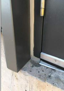
Photo 10 WIP of painting at door on right, sealant & IMP flashing on left.
