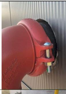
Photo 13 Sprinkler pipe penetration to be fully sealed and insulated from both interior and exterior. Clean IMP of all marks and debris.
