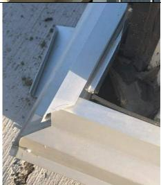
Photo 42 View looking North at NW mullion and sealant installation status. Ensure all corners are tight & caps are installed square.
