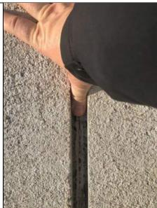
Photo 53 Sawcut grooves in drive-in ramp approx. 1x1" in size.
