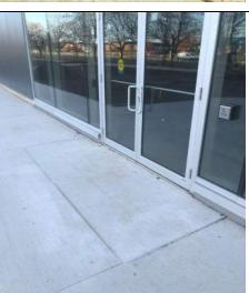
Photo 43 View looking North at NW office entrance. Sidewalk poured around frost slab pad.
