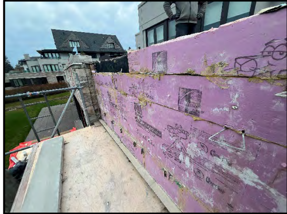
Localized removal of the stone veneer
