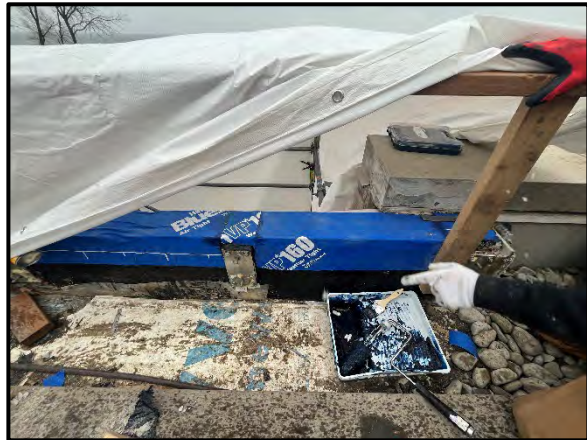
Installation of new weather resistive barrier (Blueskin VP160) along related portions of the interior knee wall
