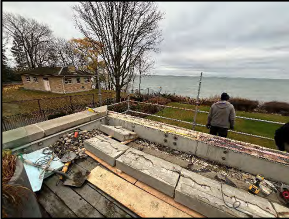
Localized removal of the coping stones
