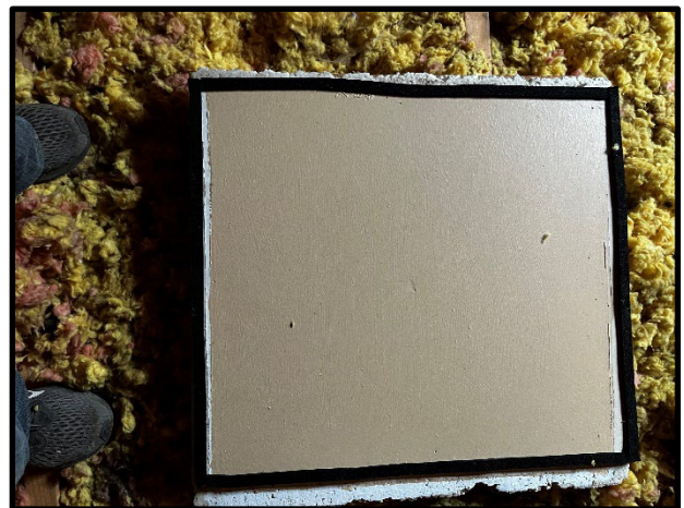
Seal attic hatch covers with adhesive backed foam gasket at Units 4-8
