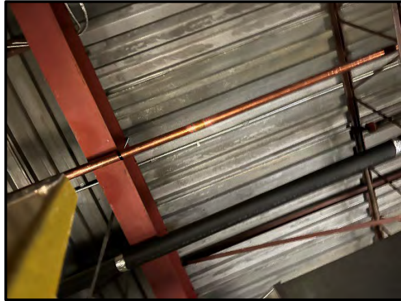
Installation of new copper DCW piping.
