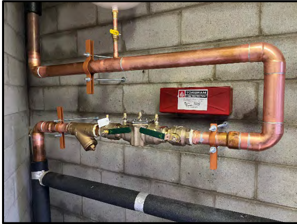
Installation of new backflow preventers
