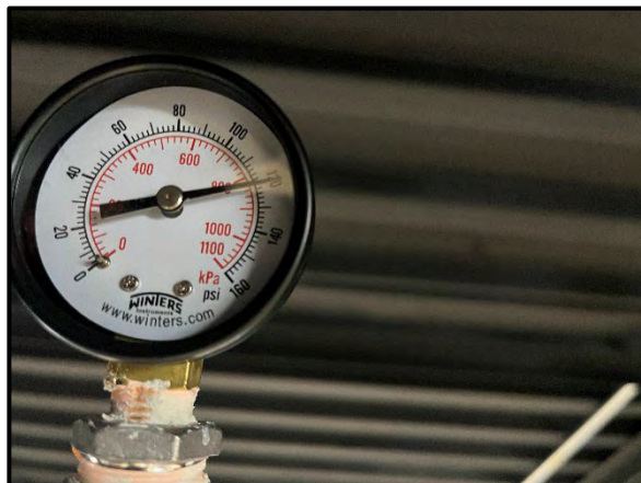
Air and water pressure tests.
