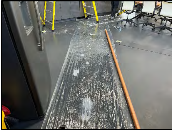
Contractor mobilized to the site.
