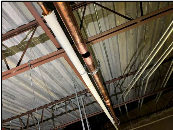
Installation of new hangers.
