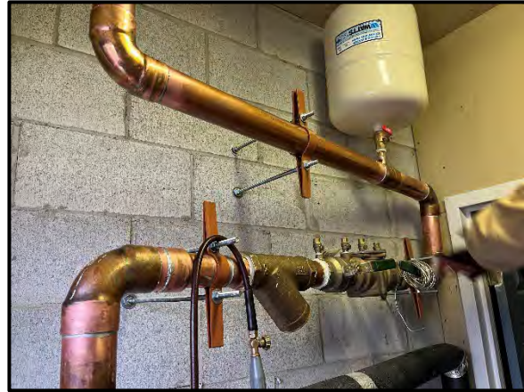
Installation of new expansion tanks.
