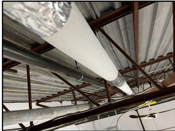
Installation of new pipe insulation.
