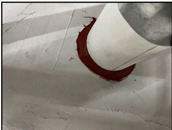
Installation of new fire-rated sealants.
