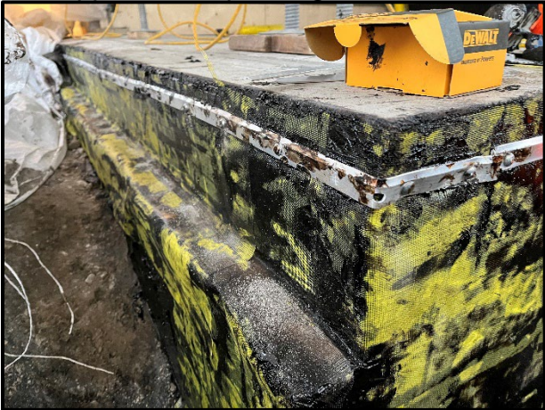
Installation of termination bars over the new cold-applied waterproofing
