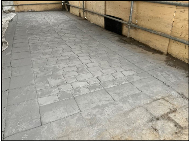
Installation of stamped concrete
