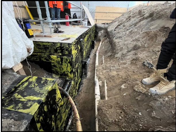
Installation of new PMMA-based waterproofing
