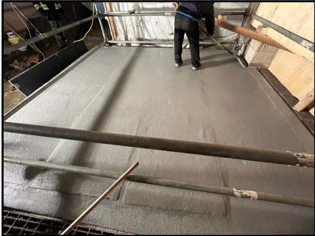
Installation of new PMMA-based waterproofing
