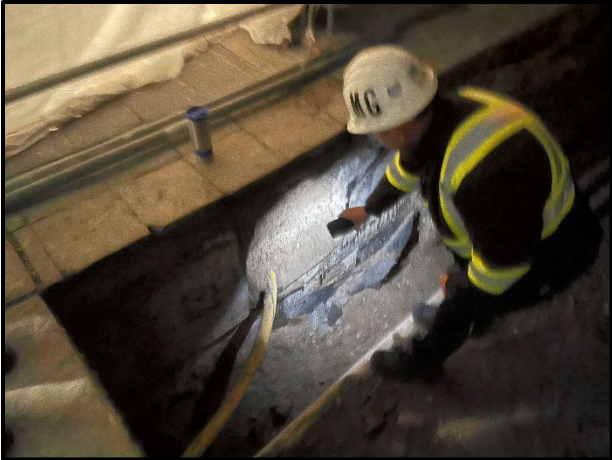
Removals along the northside of the electrical room
