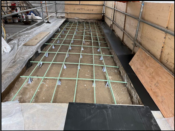
Installation of epoxy-coated reinforcement bars
