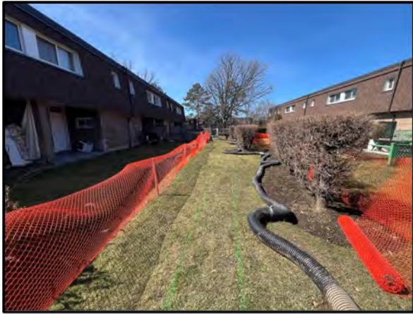
The Contractor mobilized to the site.
