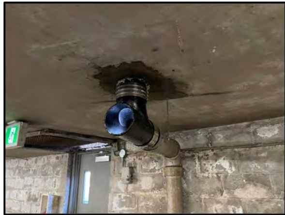
Installation of new garage roof slab drain.
