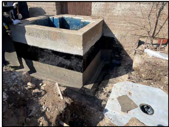
Localized repairs to garage roof slab waterproofing.
