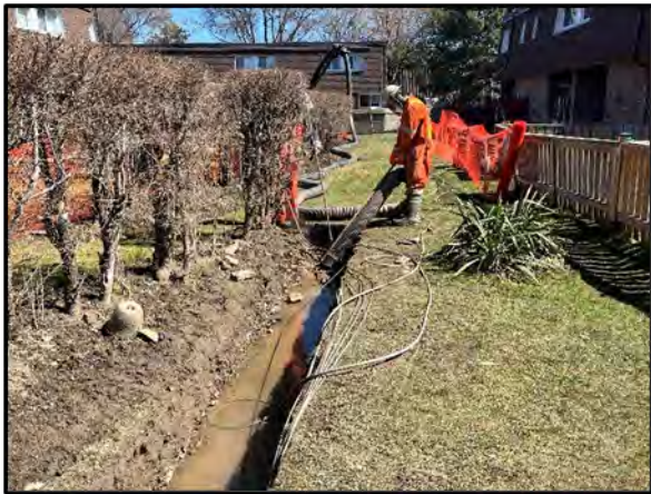
Removal of overburden materials for French Drain.
