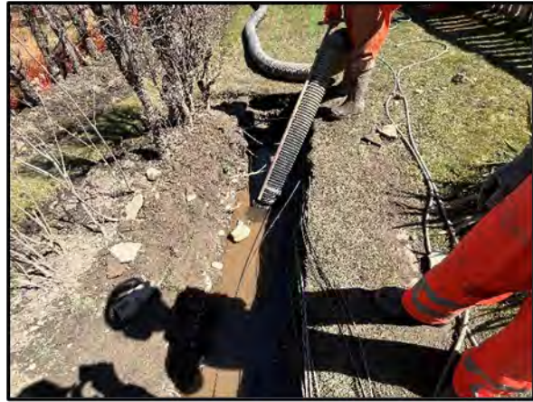
Removal of overburden materials.
