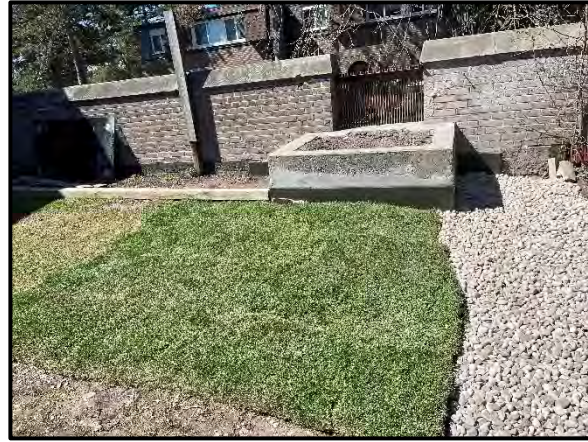
Localized replacement of deteriorated bricks. Reinstatement of overburden materials.
