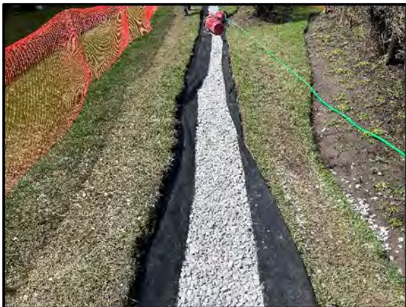
Installation of the new French drain.
