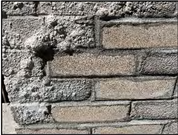
Localized replacement of deteriorated bricks. Reinstatement of overburden materials.
