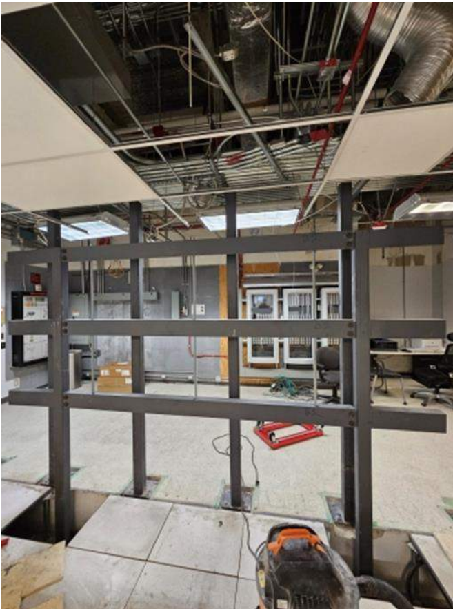
Figure 1 - Framework for Screen Monitor under Construction
