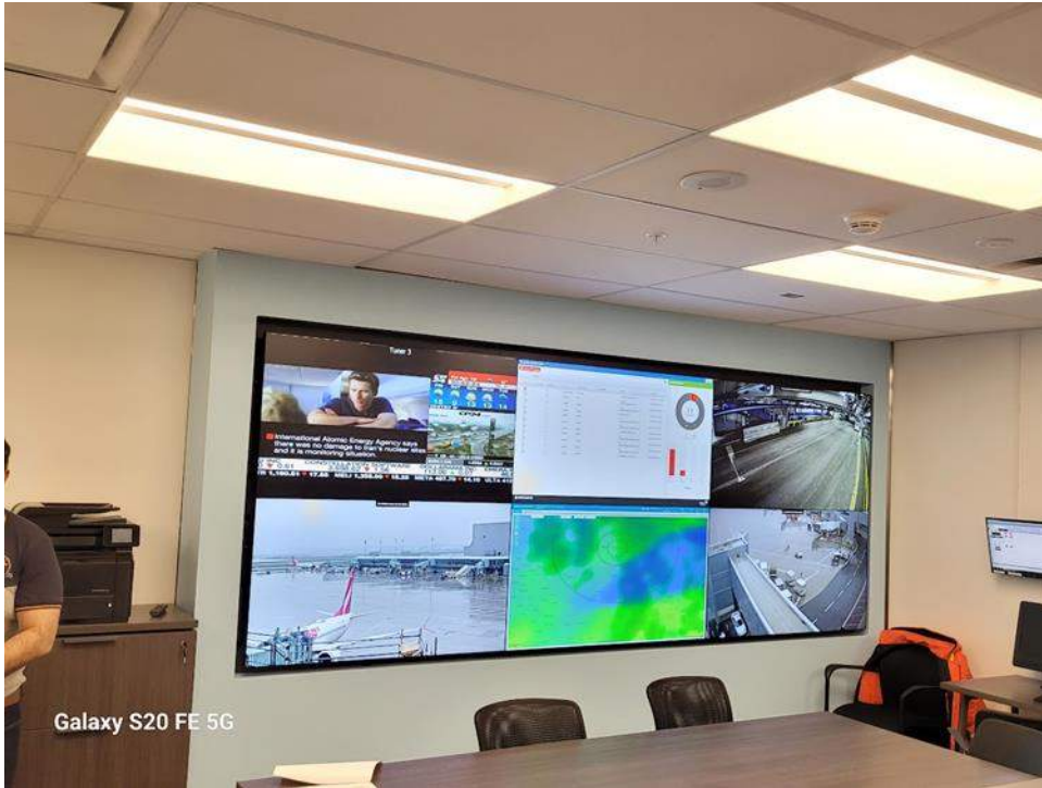
Figure 4 - Current Condition of Screen Monitor in BMS Office
