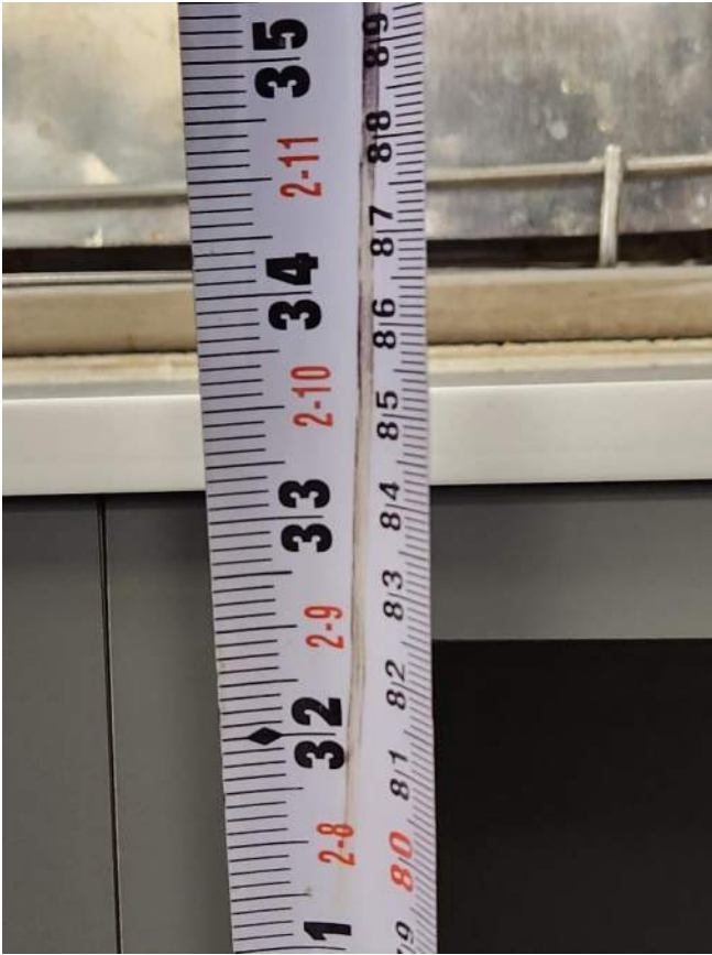
Figure 13 - Height of countertop from floor finish level was measured at: 850 mm, drawing shows height as: 860 mm.
