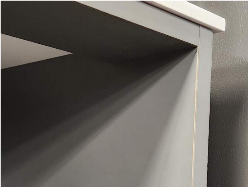
Figure 15 - Solid surface countertop protrudes beyond edge of kitchenette millwork.
