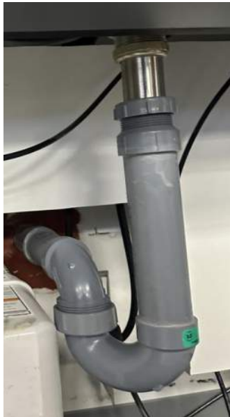
Figure 22 - Installed P-Trap
