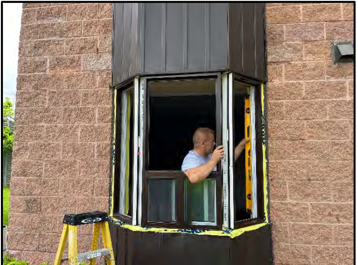
Alignment of new aluminium framed assemblies at unit 108
