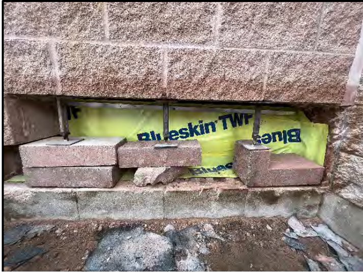
Installation of membrane flashing
