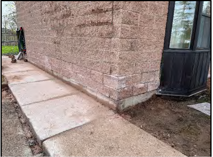
Installation of concrete blocks along the ground level
