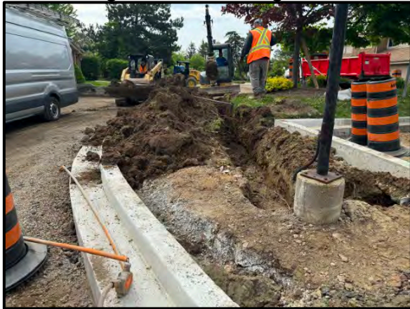
Trenching for new street light conduits.
