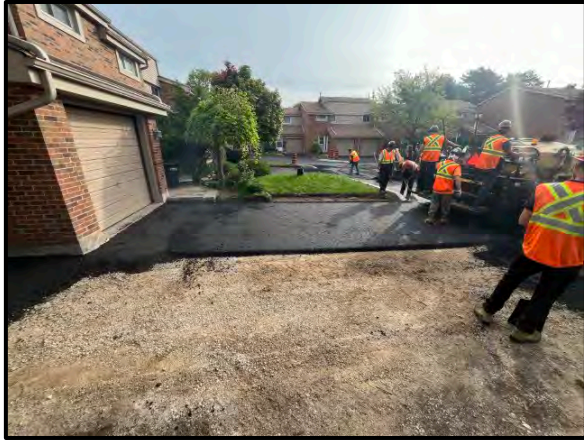
Installation of new asphalt pavement surface course.
