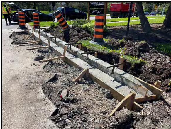
Installation of new concrete curbs.
