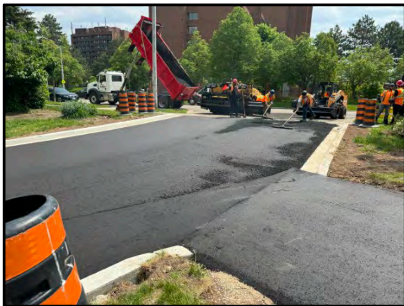
New asphalt pavement surface course.
