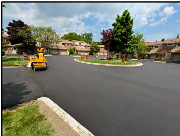
New asphalt pavement surface course.
