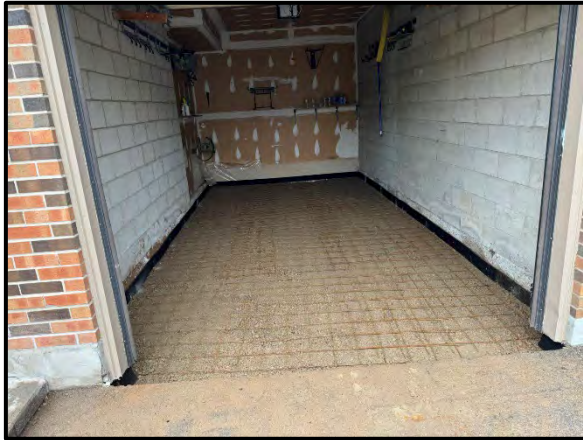
Installation of new concrete garage floor slab-on-grade within Units 25 & 31.
