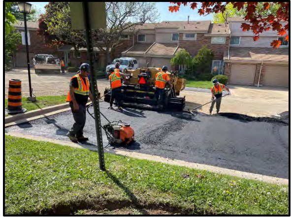
Compaction of asphalt pavement surface course.
