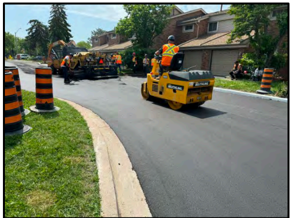
New asphalt pavement surface course.
