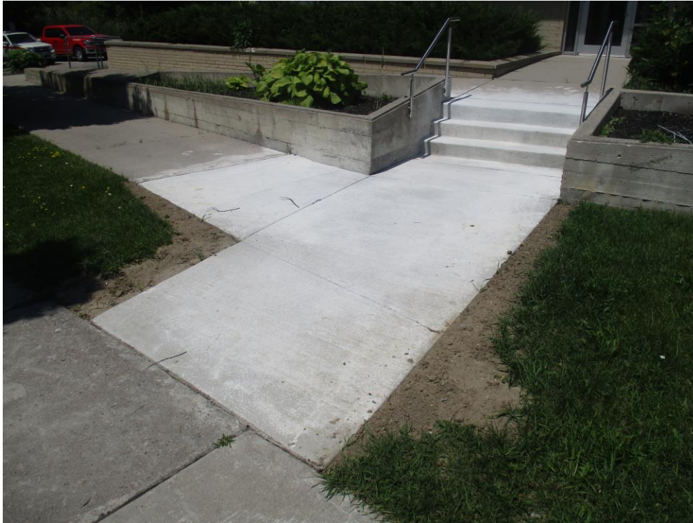
Photo 1: Damaged concrete sidewalk for area#4 has been removed and replaced.
