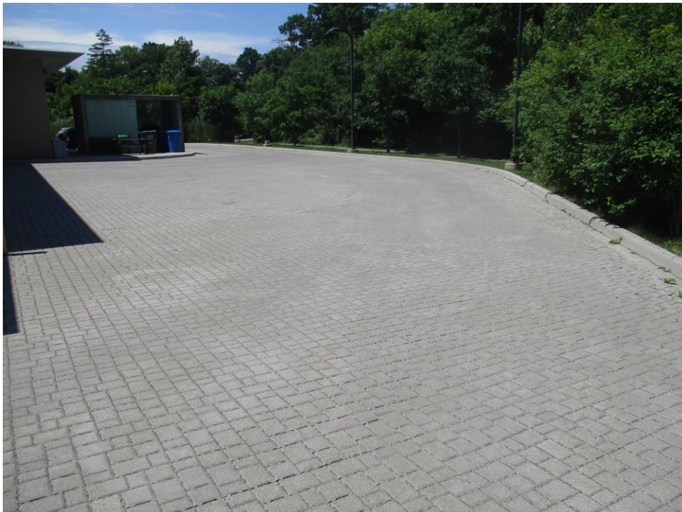
Photo 4: Joint fill material was in place between the interlock gaps at the whole areas not being releveled and reinstated.
