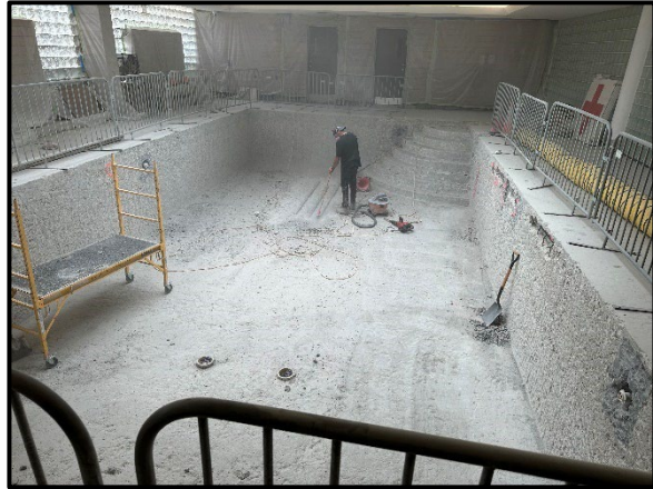
Removal of existing pool waterproofing.
