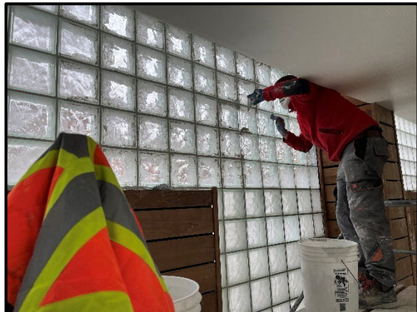
Replacement of glass block walls within the pool room.
