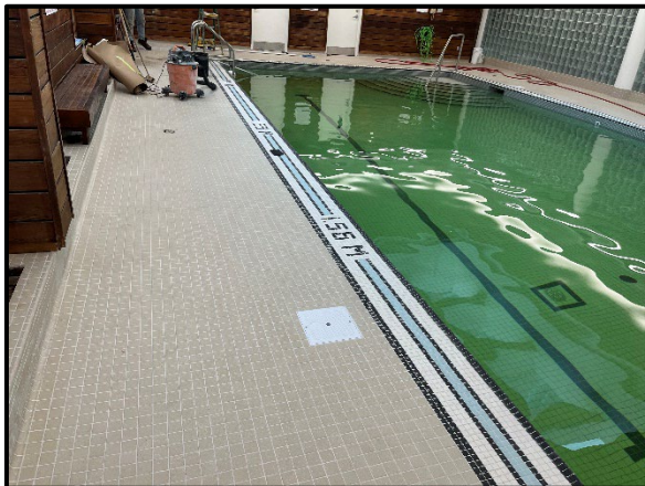
Installation of new tiling within the pool room.
