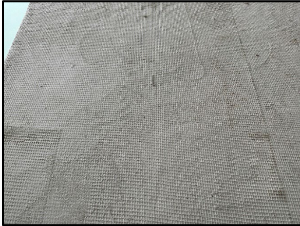
Installation of new waterproofing within the pool.
