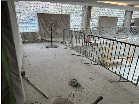
Removal of existing pool room tiling.
