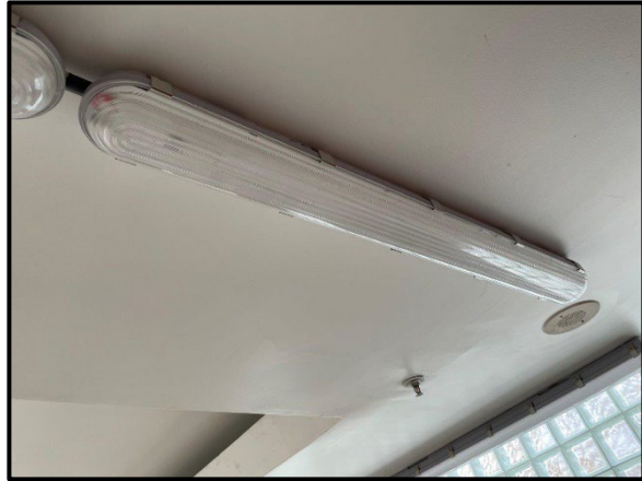
Installation of new lighting within the pool room.
