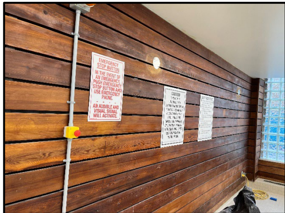
Cedar wall panelling refinishing.
