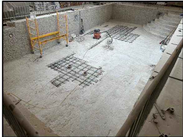
Removal of deteriorated concrete within the pool room.
