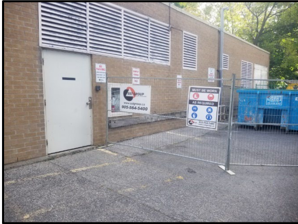
The Contractor mobilized to the site.
