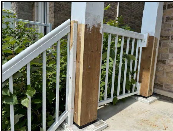
Installation of New Cladding
