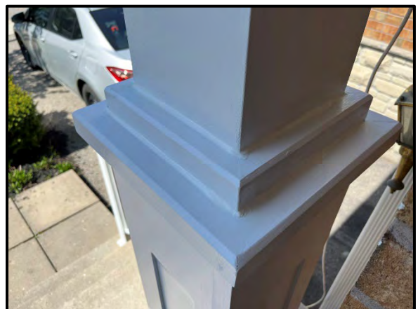
Installation of Cladding Panel Trim
