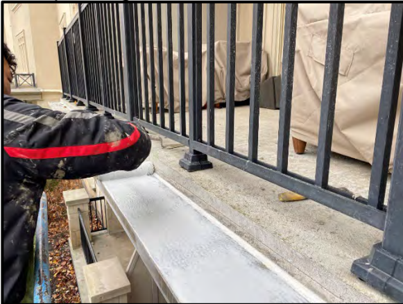
Installation of architectural coating on the exterior face of cornices
