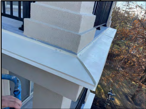
Installation of cornice flashings
