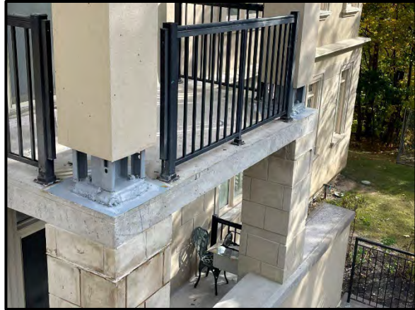
Balcony Column Base Repairs
