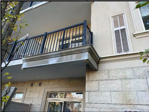
Installation of base coat of elastomeric waterproofing
