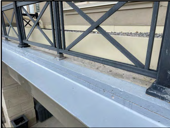
Installation of architectural coating on the exterior face of cornices
