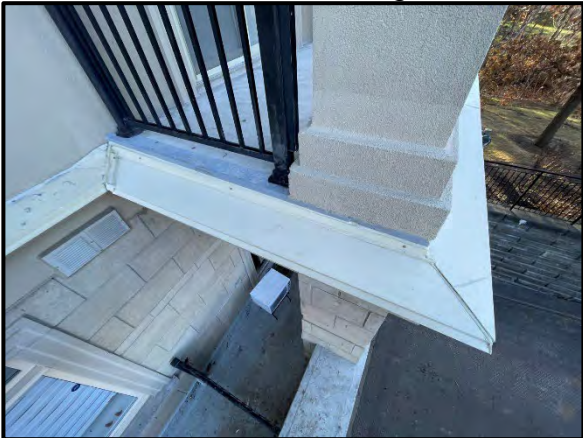
Installation of cornice flashings
