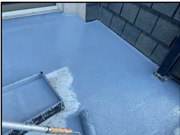
Installation of elastomeric waterproofing at 4 th floor balconies
