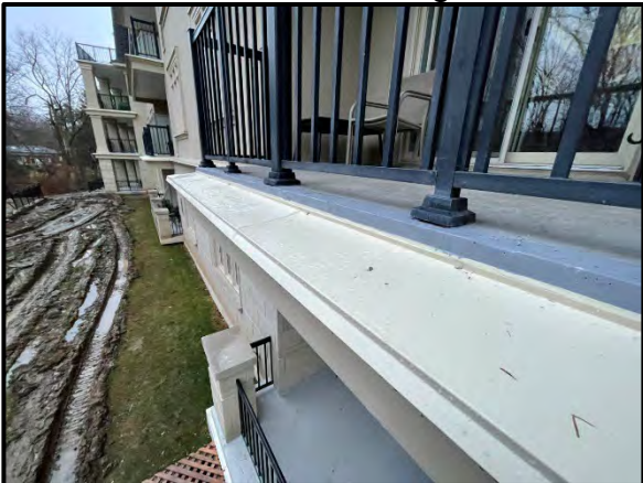
Installation of elastomeric waterproofing at 4 th floor balconies
