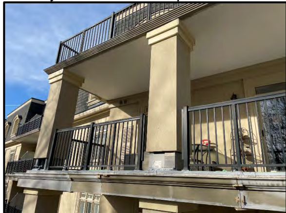
Balcony Column Base Repairs
