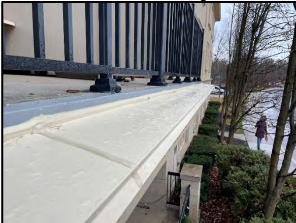
Installation of elastomeric waterproofing at 4 th floor balconies
