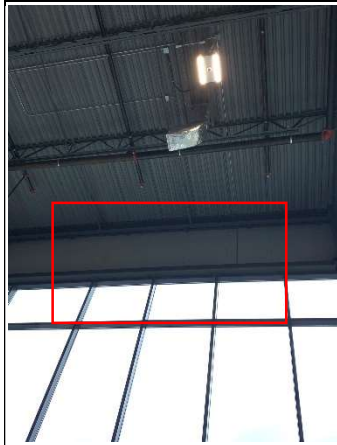
49. Scratches observed on the IMP panel on top of the mullion
