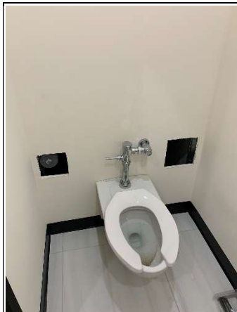
35. Missing access panel
