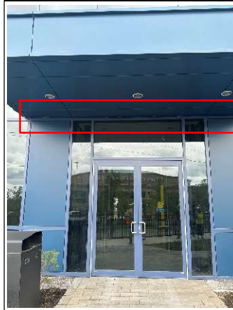
82.Gap observed between the office entrance canopies and mullions
