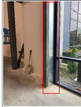
44. Installed aluminum panel between column and mullions needs to be painted to match
