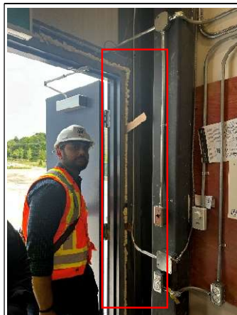
75.Foam around the electrical room door needs to be cut and caulked properly
