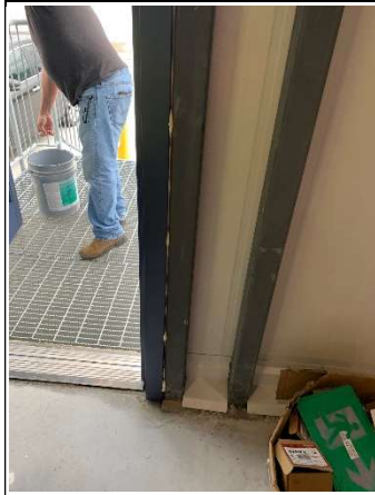
40. Caulking needed around the doors.
