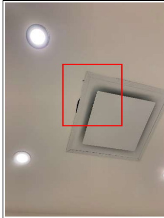
34. Patching needed around washroom grill
