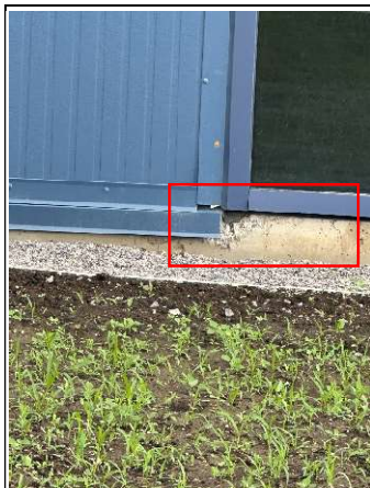
83.The outside concrete curb was damaged and needs repair work
