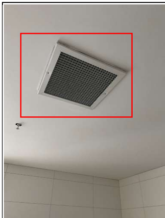
73.Caulking needed around the washroom exhaust
