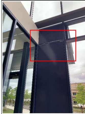
50. Vapor barrier needs to be cut and the mullions need cleaning
