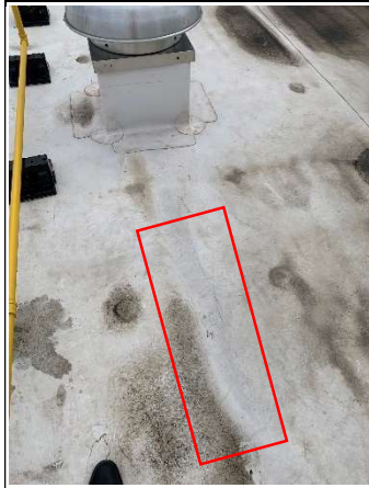
94. Air buildup observed in roofing membrane
