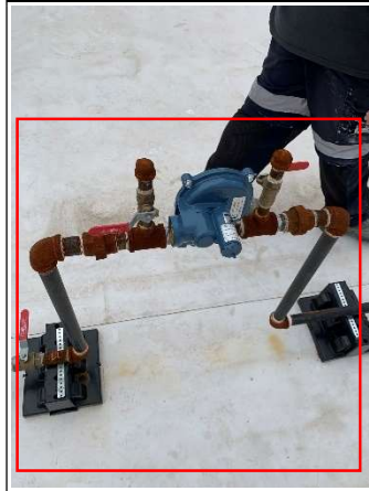
95. Rust observed in some pipes and elbows
