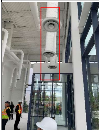
70.Ducts in the office area need alignment
