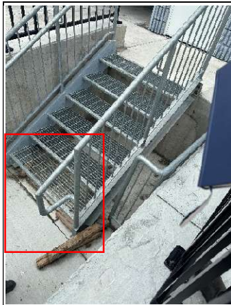
89.Stairs leading to existing building need safe installation
