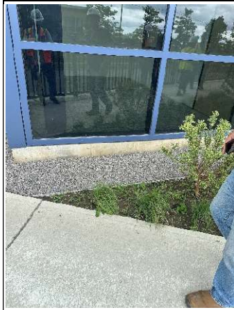
77.Missing flashing beneath the mullions
