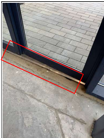
45. South door transition needs replacement
