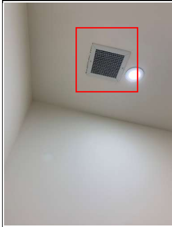
34. Patching needed around washroom grill
