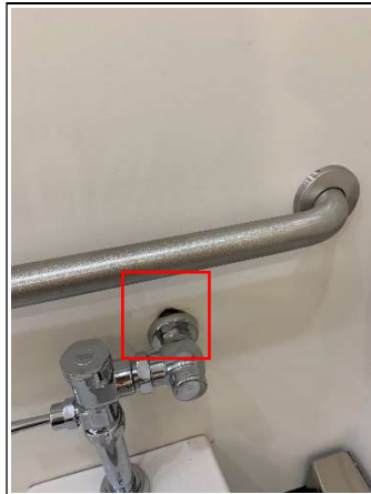
30. Patching needed around the toilet
