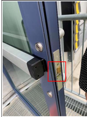
56. Door latch needs adjustment
