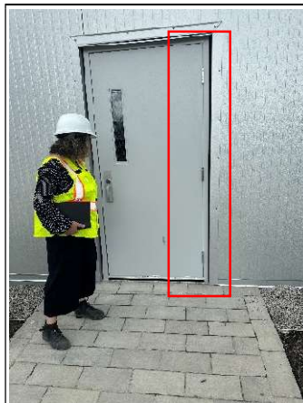
84.Caulking needed around the exit doors
