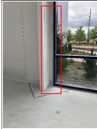
68.Foam around the mullion needs to be cut properly
