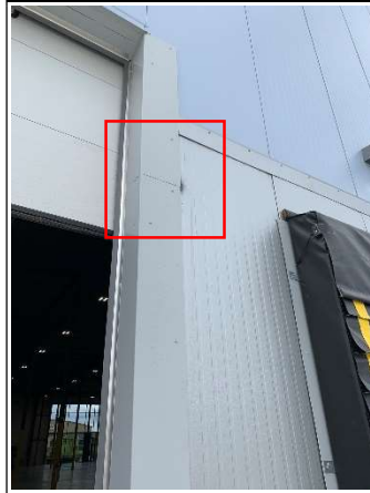
78.Paint observed on some outside panels; cleaning needed
