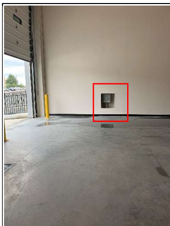
57. Access panel needed to cover the pole lighting junction
