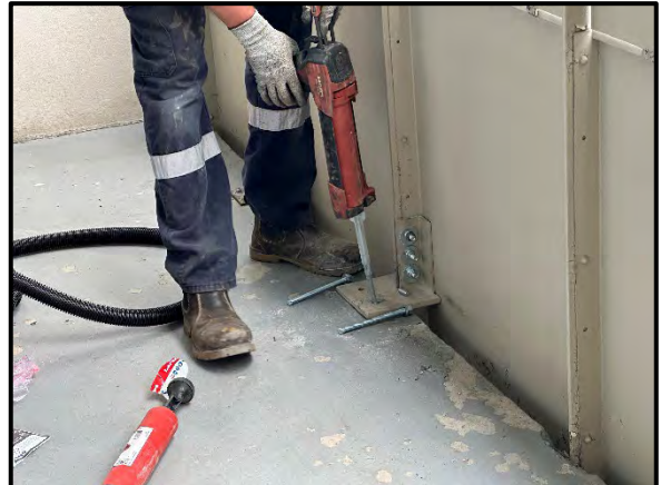
Steel Baseplate Installation
