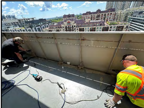
Steel Baseplate Installation
