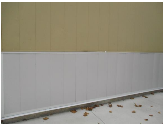
Photo #3- New metal cladding has been installed.
