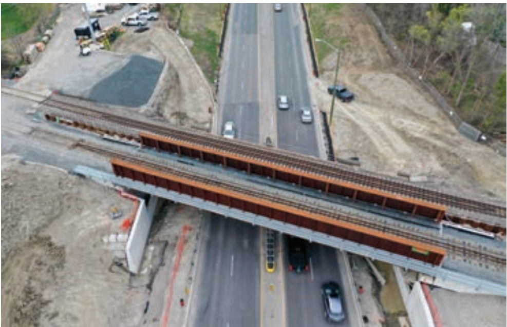
REGION OF YORK The Highway 27 and CP rail bridge taken April 26, 2021, the day before train traffic was switched over onto the new south bridge.
