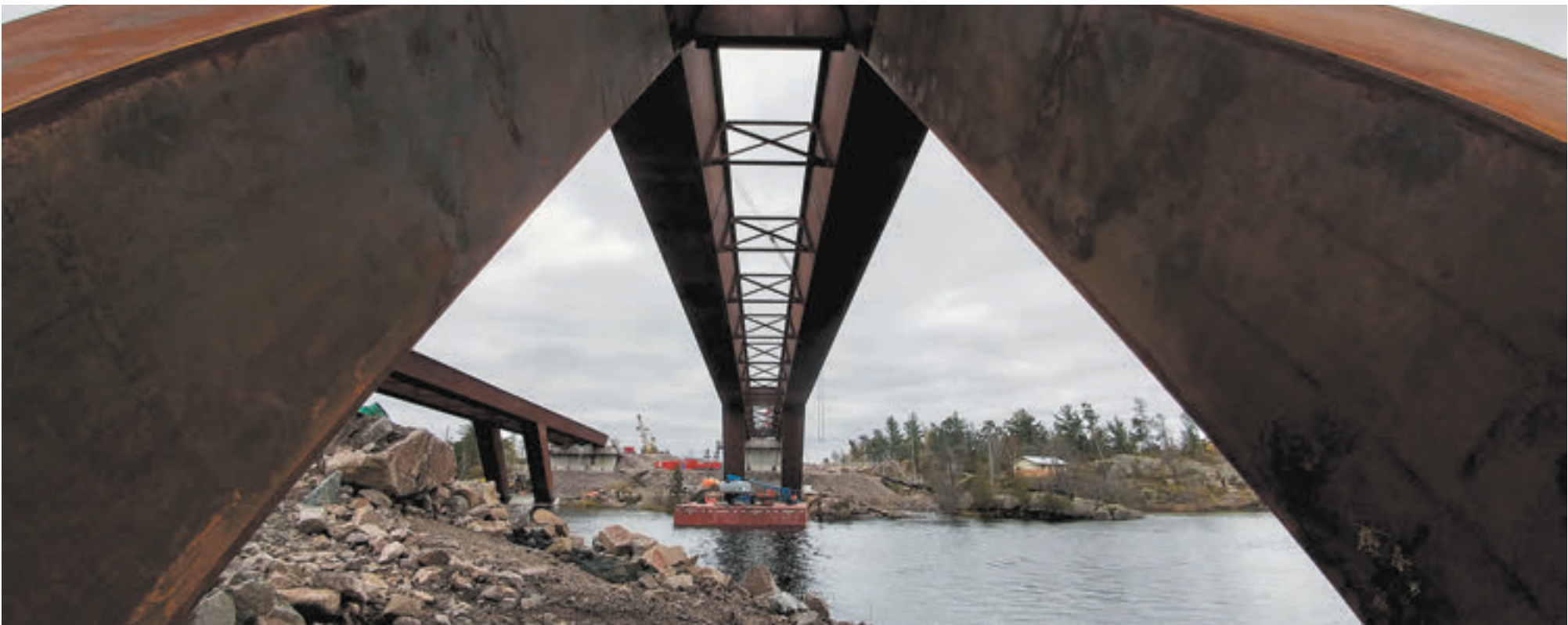
A closer look at one of the two new steel box girder bridges being built to span the Pickerel River. These leg girders weigh about 200,000 lbs. each and extend from the shoreline.
