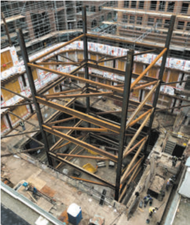
PCL CONSTRUCTORS CANADA INC. A steel shoring tower consisting of four permanent columns, along with temporary bracing that supports the heritage facade on the Two Queen Street project, was necessary due to the complexity of the project. The tower is also the permanent support for the readapted building.
