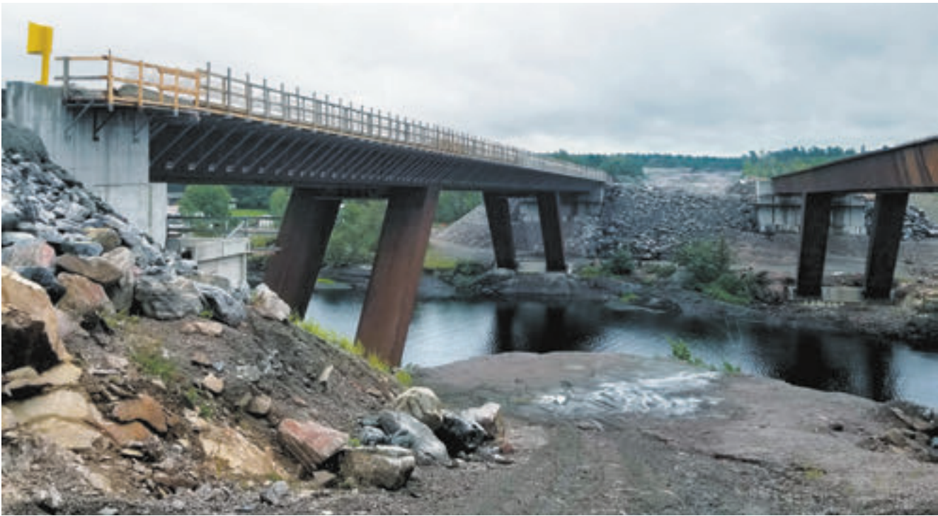
Steel was selected for the new Pickerel and French River bridges due its light weight and easier erection process for long-span bridges. The two Pickerel River Bridges (above) are 4.5 km south of the Hwy. 607 and Hwy. 69 junction.
