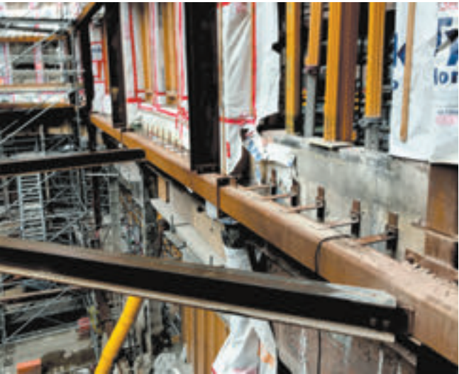
PCL CONSTRUCTORS CANADA INC. HSS walers provide a means of distributing loads from the facade to lateral braces that tie in to the steel shore tower.
