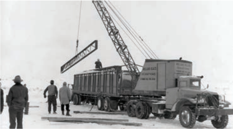
Construction of the first Canam plant in Saint-Gedeon-de-Beauce, Que., in 1960.
