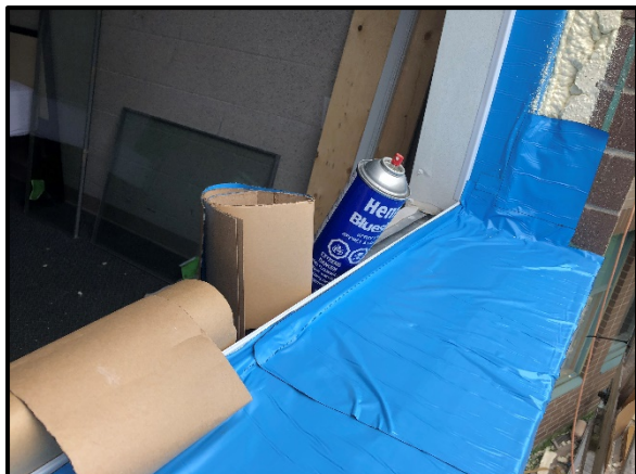
Self-Adhesive Membrane Installation
