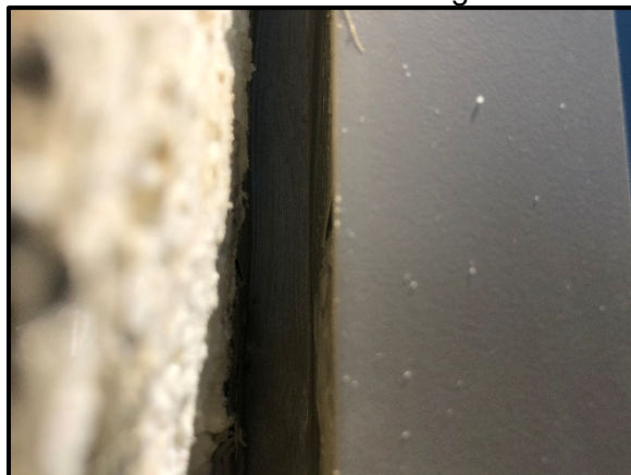
Installation of heel bead caulking
