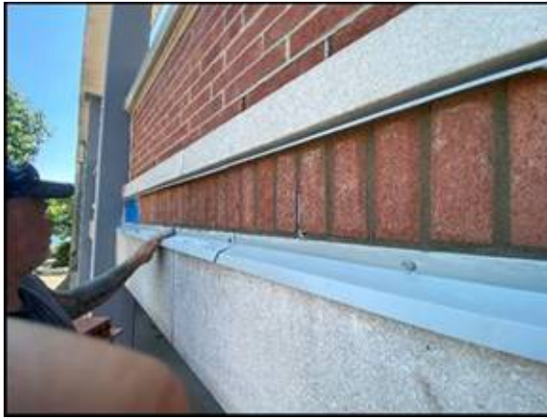
Through Wall Flashing Repairs at East Colonnade Solider Course
