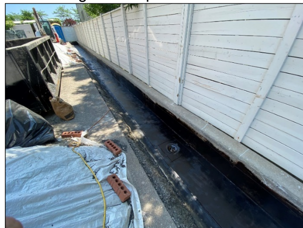
Garage Roof Slab Waterproofing Repairs West Garage Wall Upturn
