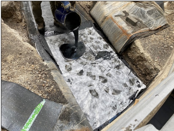
Garage Roof Slab Waterproofing Repairs Front of Building
