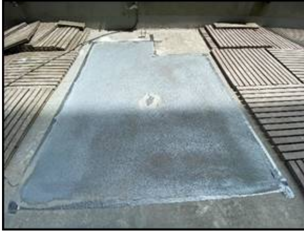
Drain Replacement and Waterproofing Repair at Unit 213 Balcony
