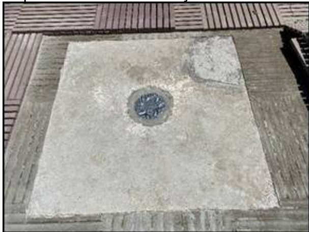
Drain Replacement and Waterproofing Repair at Unit 213 Balcony
