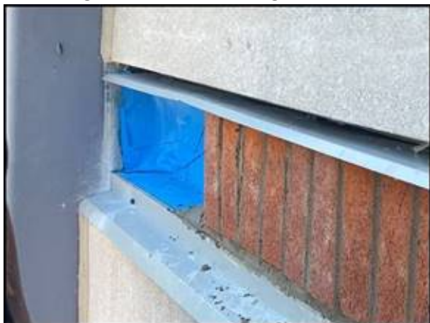
Through Wall Flashing Repairs at East Colonnade Solider Course
